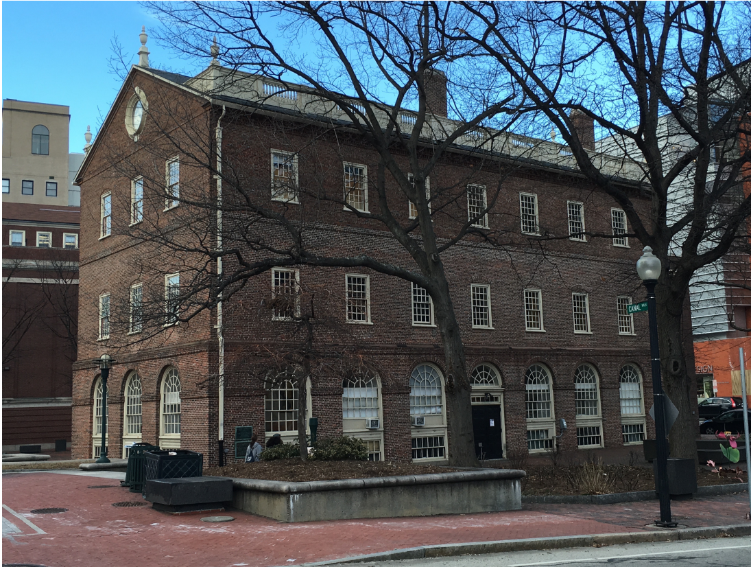
Fig. 24 The Market House, Providence RI, 1773, Joseph Brown, architect w/Stephen Hopkins. West end and south side. Photographed by Nekoro Giscombe
