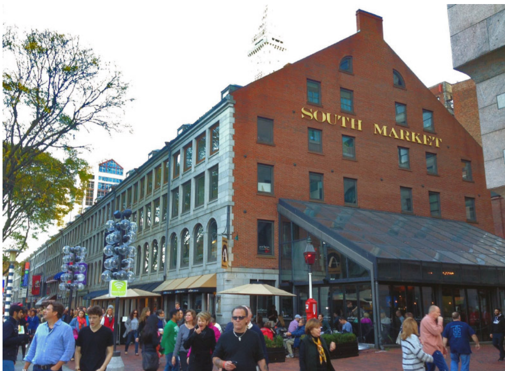
Fig. 37 Faneuil Hall Market/Quincy Market Place South Market, Boston, MA Alexander Parris, 1830-1856 Photographed by the author
