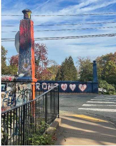
Fig. 3.2.2. Beta Bridge at UVA, column view
