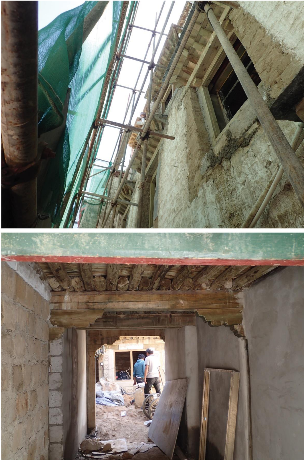
Figure 4.5. Nagtsajang Building Under Restorative Reconstruction, August, 2016.
