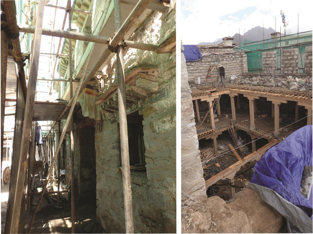
Figure 4.4. Tadongshar Building Under Restorative Reconstruction, August, 2016.
