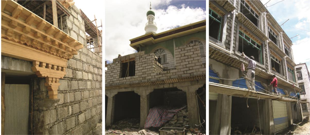
Figure 3.1. Examples of Simsha Tibetanized Construction in Lhasa: Left , Wooden shingsak (Tib. shing brtsegs ) 183 Awnings Over Entry and Standard Size Chinked Masonry on the Newly Constructed Numa House (Ka 22); center , Standard Size Masonry and Cast Concrete Traditional Tibetan Style Columns; right , Poured Concrete shingsak Awnings.
