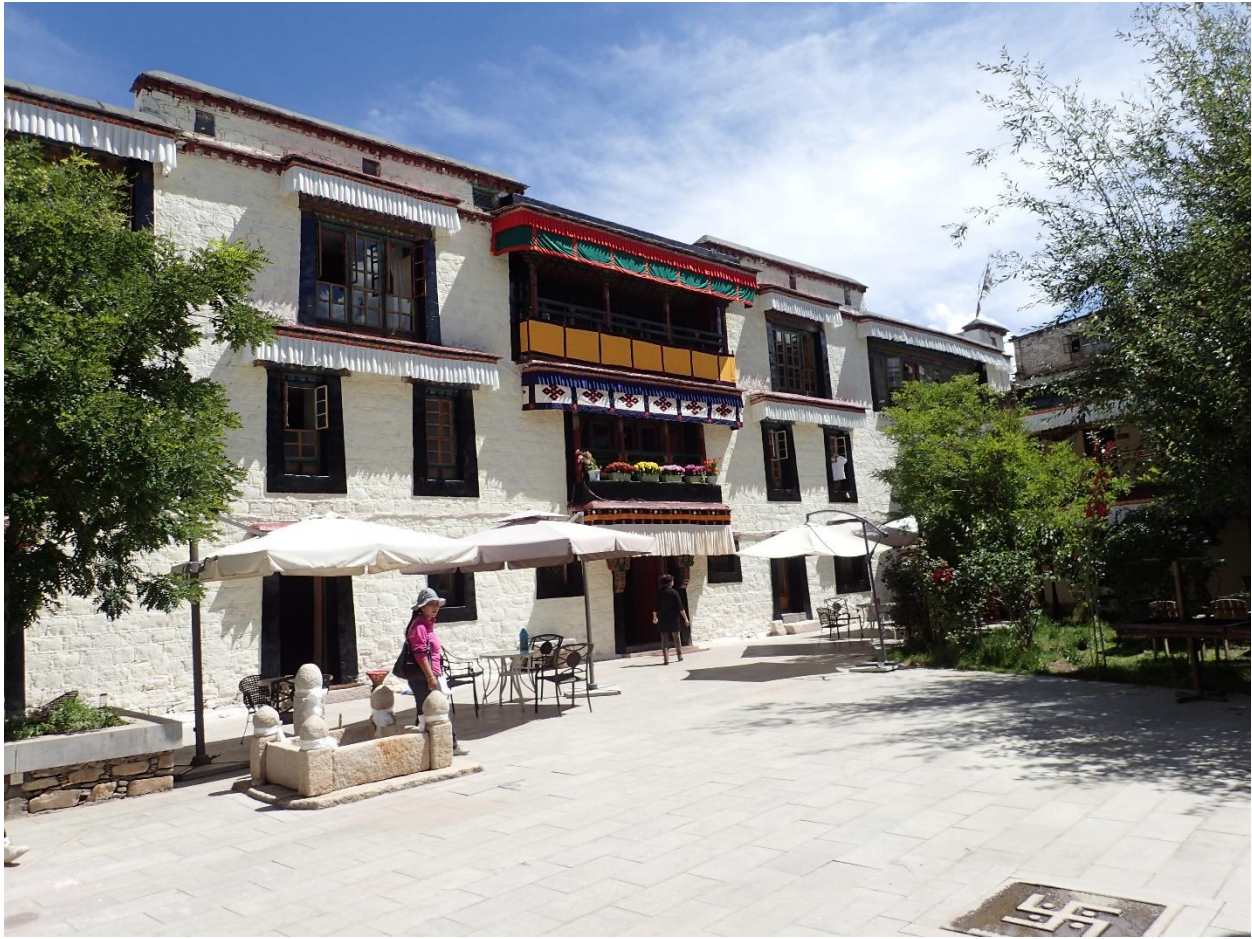
Figure 4.8. Yabshi Phunkhang, South Façade from Main Courtyard, August, 2016.
