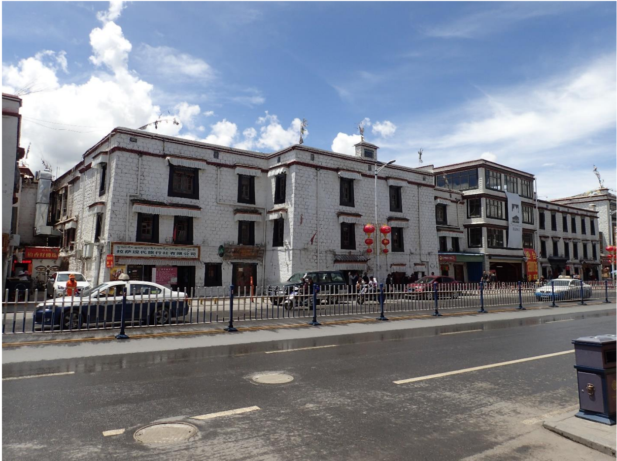
Figure 4.7. Yabshi Phunkhang, Main Façade View from Beijing Road East, August, 2016.
