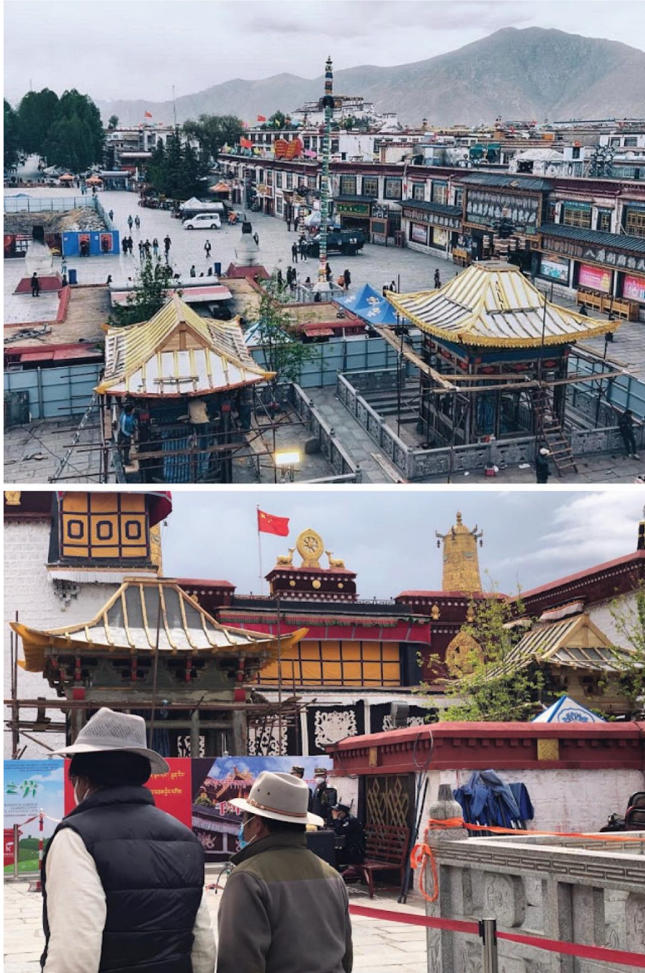
Figure 4.2. Chinese Architectural Style Housing Over the Treaty of 1821 Doring and the Princess Wencheng Willow Monuments in Front of the Jokhang Tsuklakhang. Above , Anonymous, “Two Chinese stele pavilions being built in front of the Jokhang Temple,”; below , Tsering Woesser, “Images of the Chinese-style pavilions being constructed in front of the Jokhang Temple in Lhasa, Tibet.”
