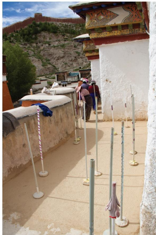
Figure 1.13. Arga Roof Stamping Dance and Babdo Stamping Tool: Above , David Germano, 2000, Arga Stammer Dance at the Jokhang Tsuklakhang; below , Will Rourk, 2016, Arga babdo Stamping Tools at Gyantse Kumbum.
