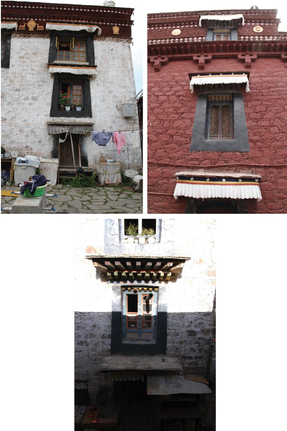
Figure 1.8. Traditional Tibetan Architectural Windows from Meru Nyingba: Above left , Windows Adorned with Textiles in the Courtyarded; right , Windows adorned with Awning Textiles on the Main North Facade; below center , Window Revealing Tsingshak Cantilevered Awning Structure.
