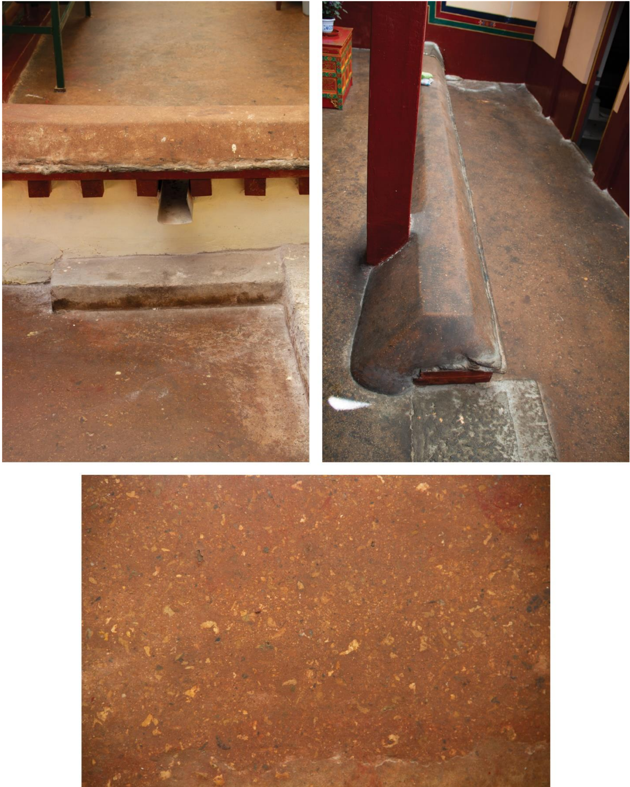
Figure 1.12. Traditional Tibetan Argas Roof and Floor Surfaces at Yabshi Phunkhang.
