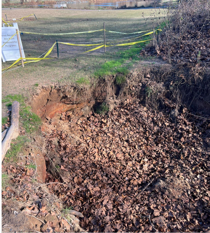
Figure 3: Status of head cut from November 26, 2024
