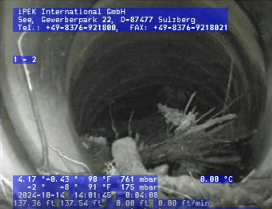
Figure 7: Footage of Blockage Within Existing Pipe
