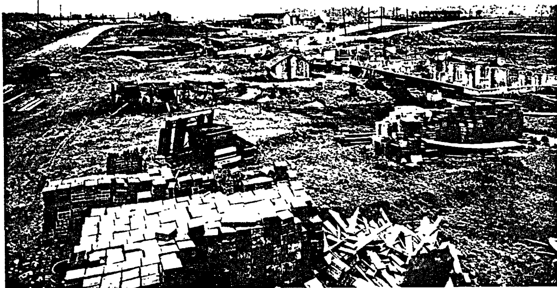
Fig. 41. Building operations, Forest Hills Inn, November 1910. The small building in the distance (above center), was probably the temporary factory established for construction of the concrete panels.
