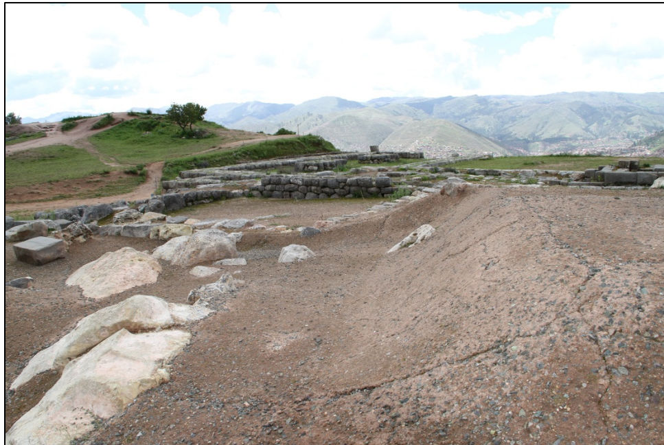
Figure 2.9: Impermeable clay cover above the third wall (Miksad)
