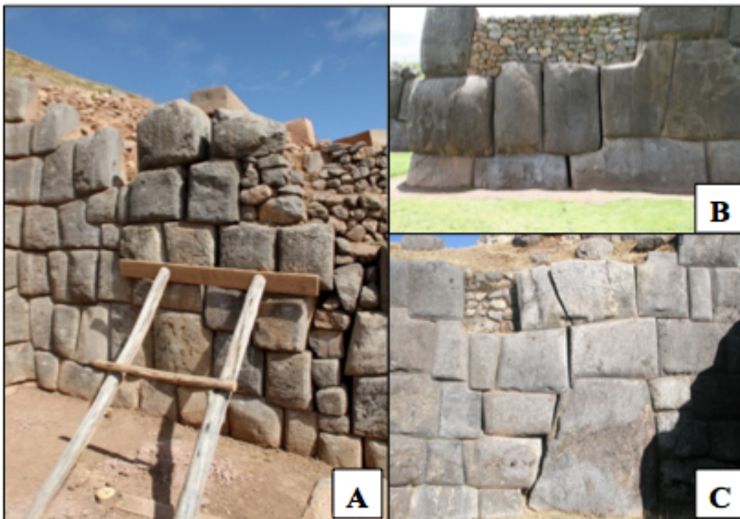
Figure 3.1: Physical evidence of damage to the third Great Wall due to hydrostatic pressure build-up: a) Support structures needed for bulging walls; b) Separation of stones; c) Vertical shearing (Miksad)
