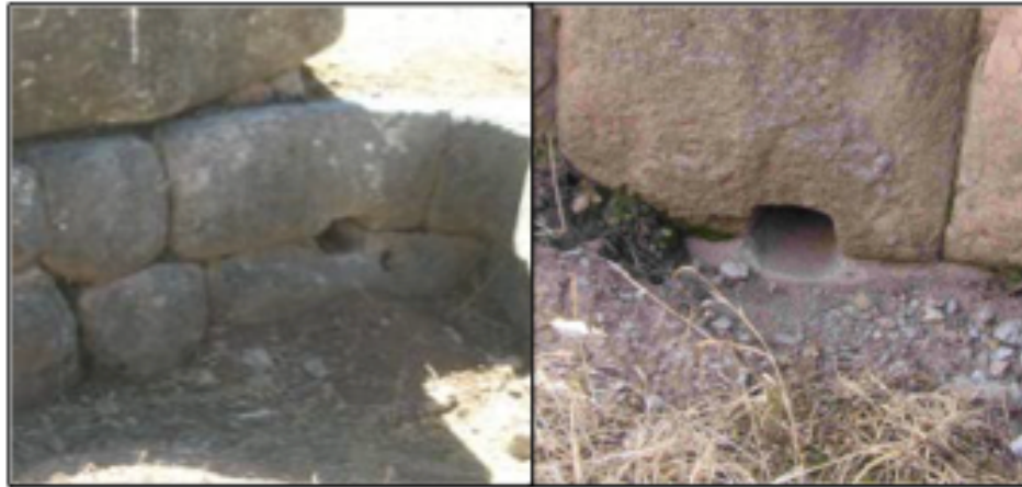
Figure 3.2: Examples of drainage ports in the second Great Wall (Miksad)
