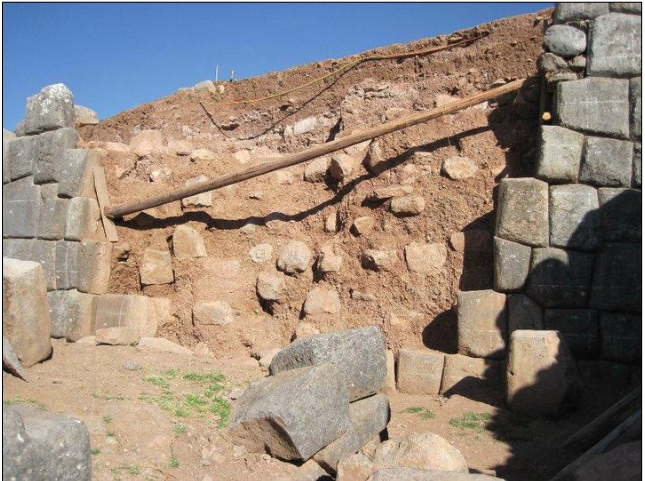
Figure 1.3: Collapsed section of the third Great Wall (Wildfire et al., 2011)
