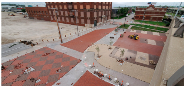
Permeable pavers near I-670 and Liberty Street allow rainwater to soak into the ground and also create a public event space.
