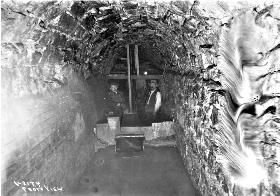
Figure 9. Underground construction of sewer at OK Creek and Main Street around 1910. Courtesy of Missouri Valley Special Collections, Kansas City Public Library.
