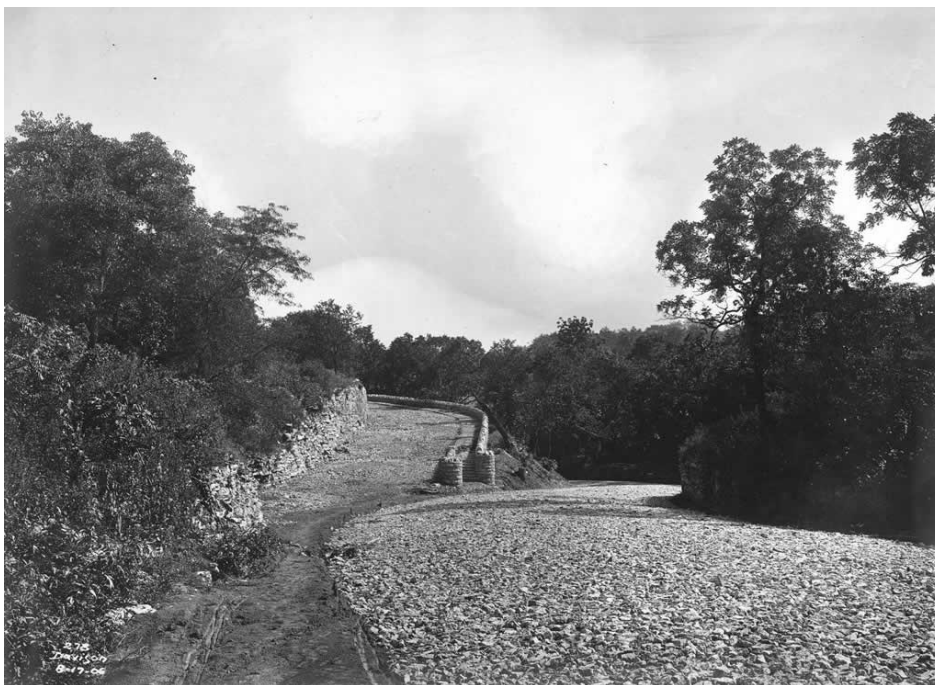
Figure 18. "Looking Northeast near 37th and Wyoming, 1906. Road surfacing in progress." Courtesy of Kansas City Parks and Recreation Archives, P-R3-001. Accessed through Roanoke Park website's "Historical Photo Gallery" webpage.
