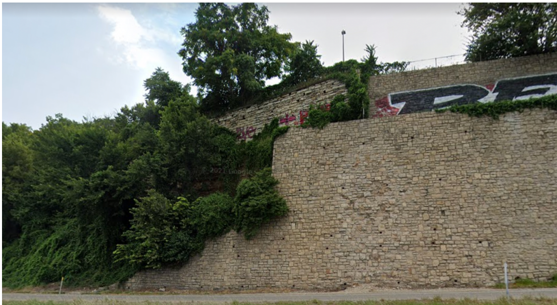
Figure 32. Intersection of early 20 th -century walls of West Terrace Park and modern walls alongside I-670, which now show signs of crumbling.
