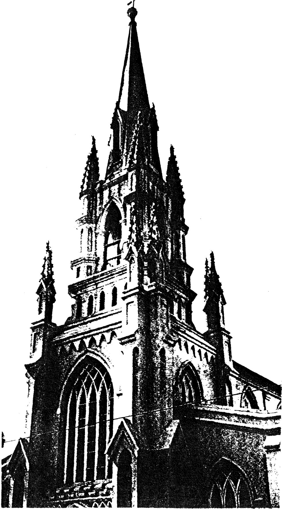
49. Grace Episcopal Church, Charleston, S.C. Exterior, tower.
