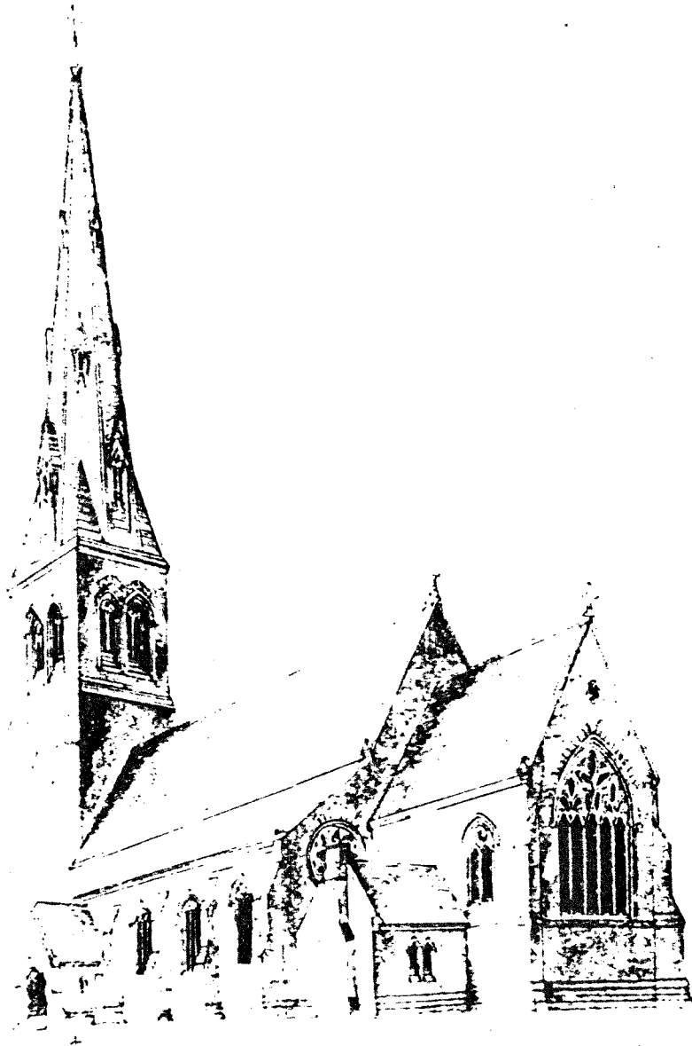
6. St. Oswald's, Liverpool. 1839-1842. A.W. Pugin. Southeast view.
