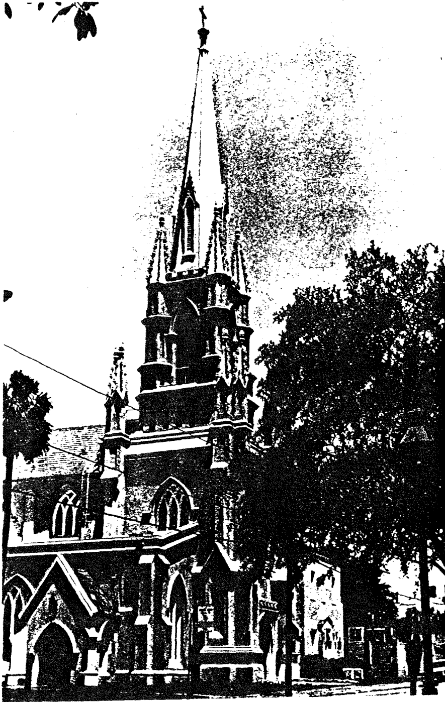
44. Grace Episcopal Church, Charleston, S.C. Exterior, view of tower with pinnacles.
