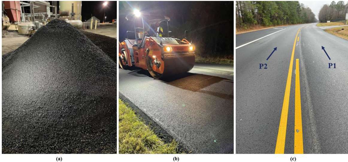
Figure 4. (a) Loose RPM Asphalt Mixtures, (b) RPM Pavement Being Compacted, (c) RPM Pavements in-Service 4 Months After Placement on Old Stage Road in Chesterfield County, Virginia. (Virginia Asphalt Association, 2022)
