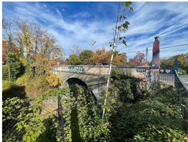
Fig. 3.2.1. Beta Bridge at UVA, wide view
