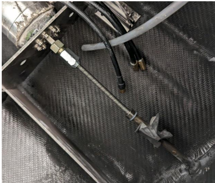
Figure 26: Flexible Shafts Installed and Connected to Motors
