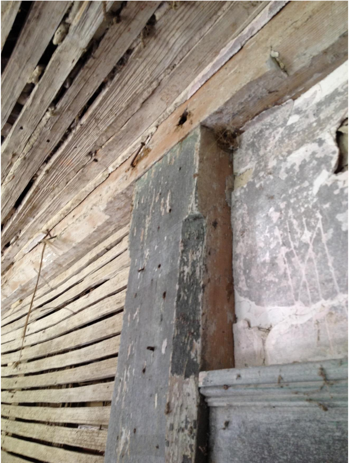
Figure 35. Detail of wall framing post and plate at Pear Valley. Note chamfers and lamb's tongue stops. Photo by author.
