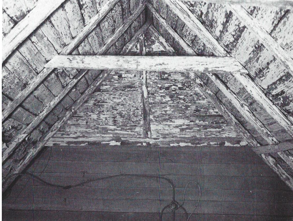
Figure 44. View of the interior of the roof of the Ball-Sellers House, Arlington County, built c. 1750-1775. Note the insubstantial riven rafters and clapboard sheathing. From Upton, Holy Things and Profane , 111.
