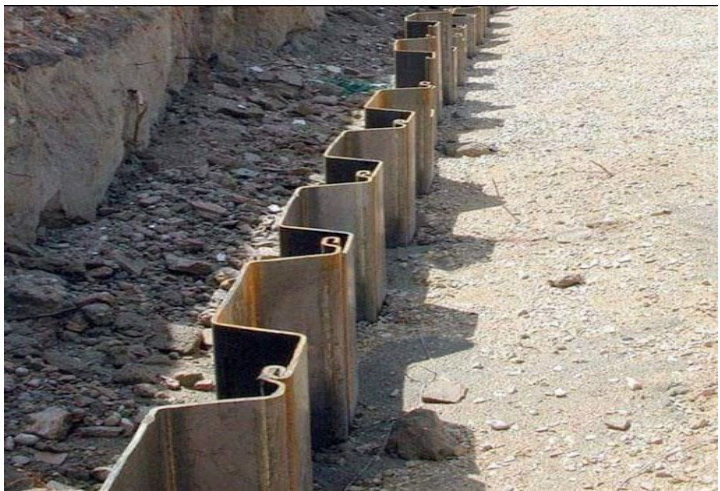
Example of sheet piles in place
