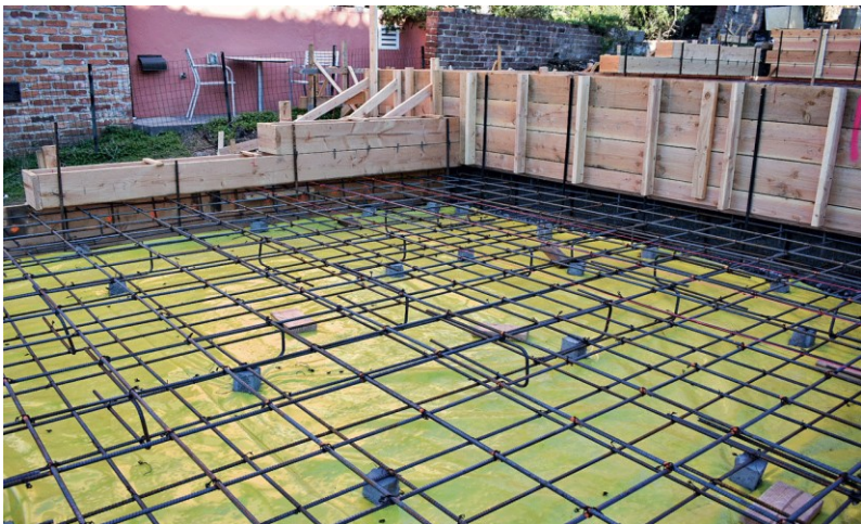
Example of Mat Slab Installation
