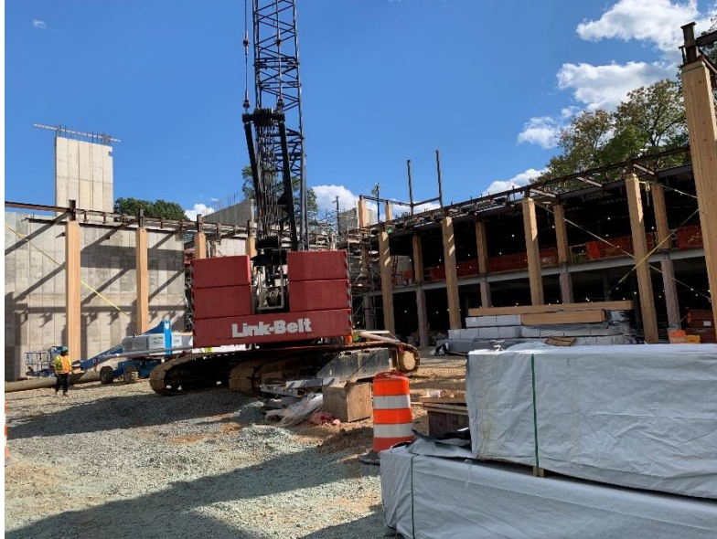
Figure 2: Inside View of the Contemplative Commons Construction Site
