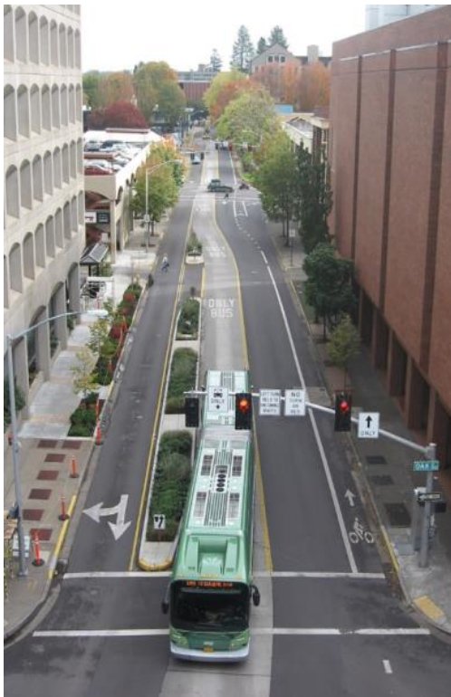
Figure 4. Partially completed BRT system in Madison, WI. (City of Madison, 2024).
