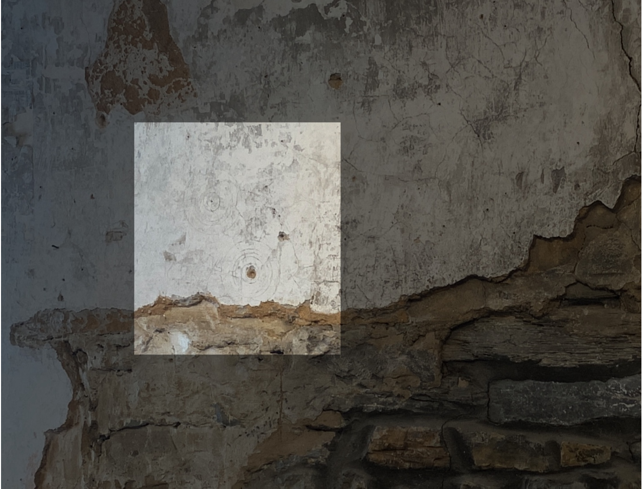
Figure 12. Historical concentric circle graffiti above hearth in Burwell-Morgan Mill. May 2023. (Photograph by Author)
