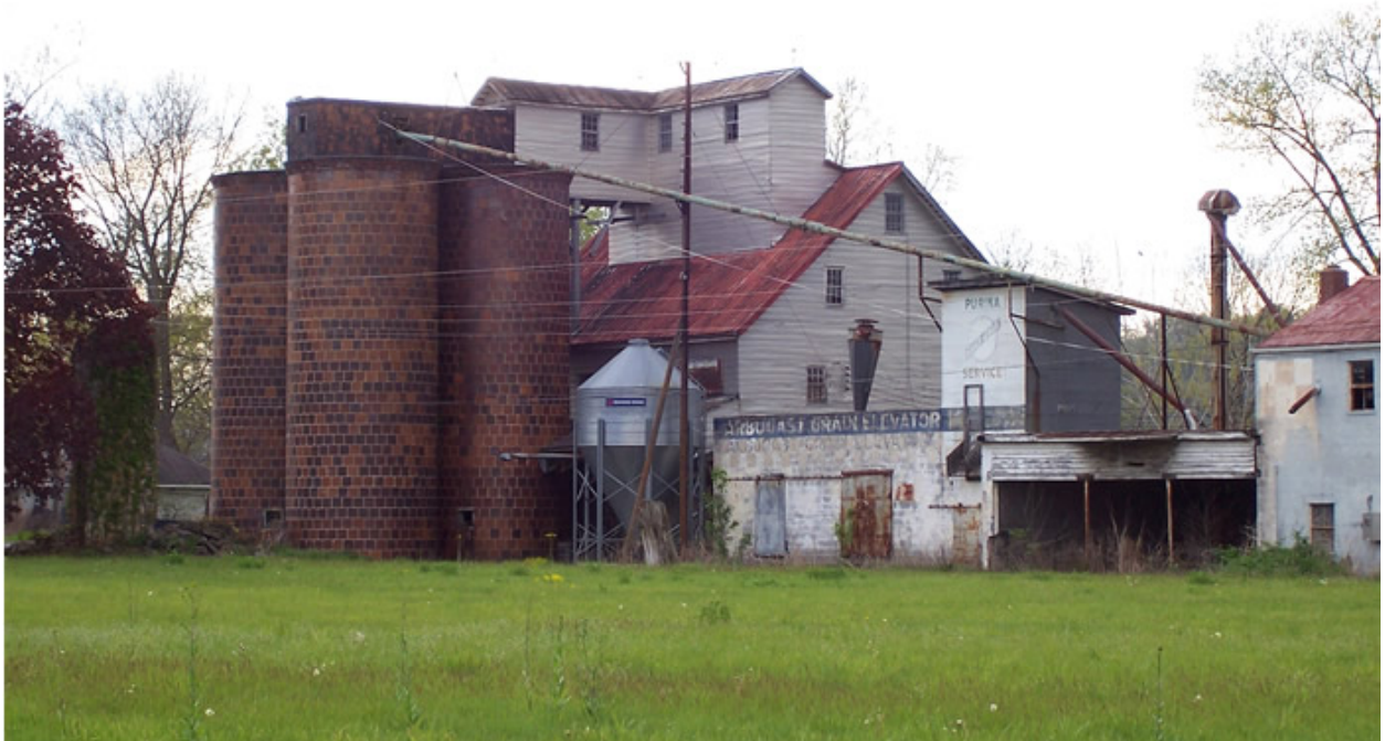
Figure 1. Photograph of the Plains Mill taken in 2005. The 19th-century core structure is visible behind the 20th-century additions. Kinsey, Robert T., "Plains Mill/Arbogast Grain Elevator" 2005, Millpictures.com, Accessed December 13, 2023, https://millpictures.com/mills.php?millid=1404
