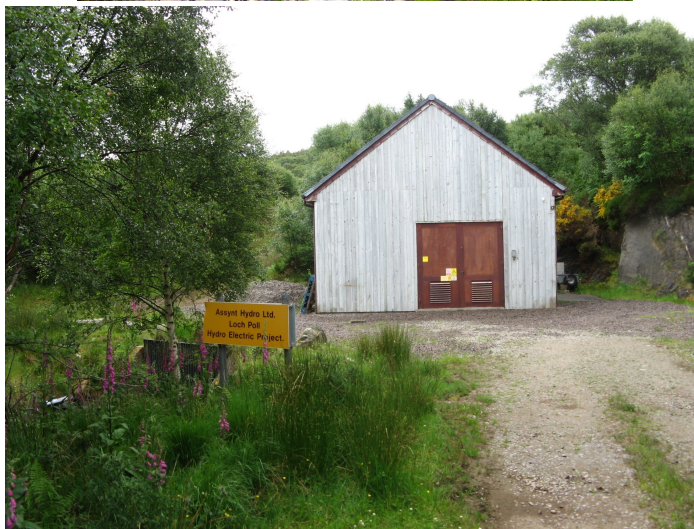
Upper (left) and lower (right) portions of hydroelectric facility owned by the Assynt Crofters Trust. If sufficient water above a minimum amount which must be maintained in the stream is available, the water is redirected through a pipe which runs along the stream downhill to the generation station below. This facility provides the Trust with its main source of financial stability.
