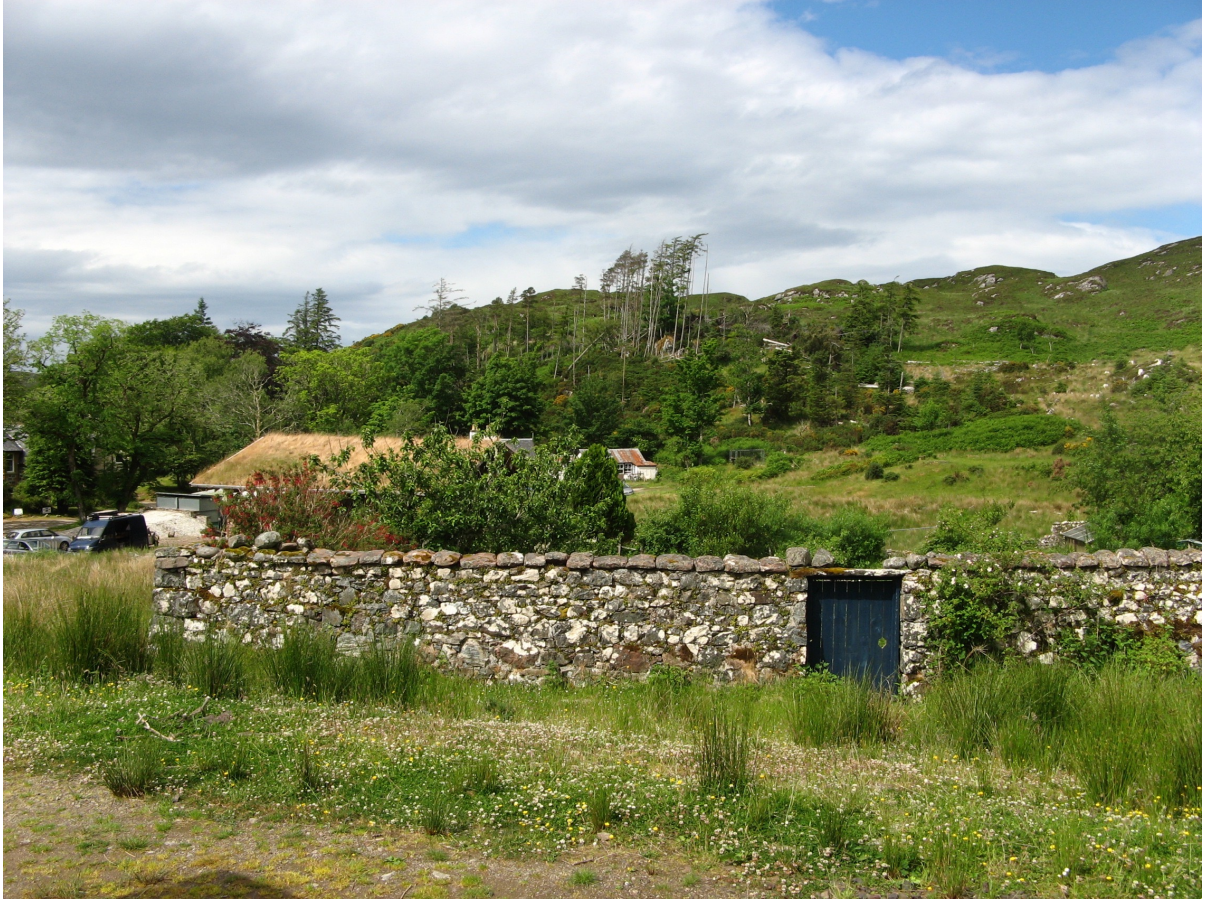
Ruined walled garden behind the lodge at Glencanisp on Assynt Foundation land. Subsequent to the taking of this photo, the garden has been restored. The green roofed pole barn is in the background.
