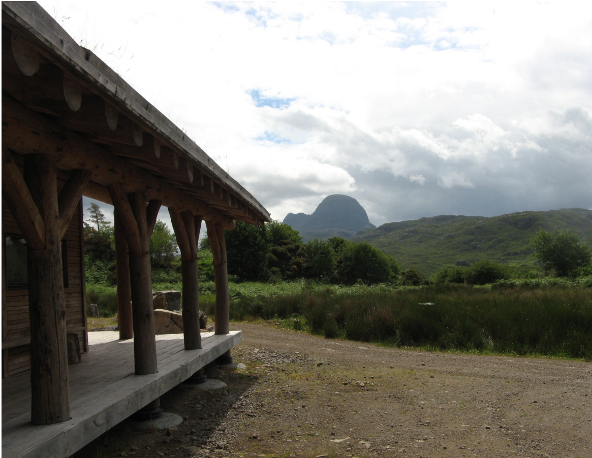
The front porch of the Assynt Foundation's Community and Arts Building, with Suilven in the background, 2016. The plants growing on the building's green roof are visible above the eaves.
