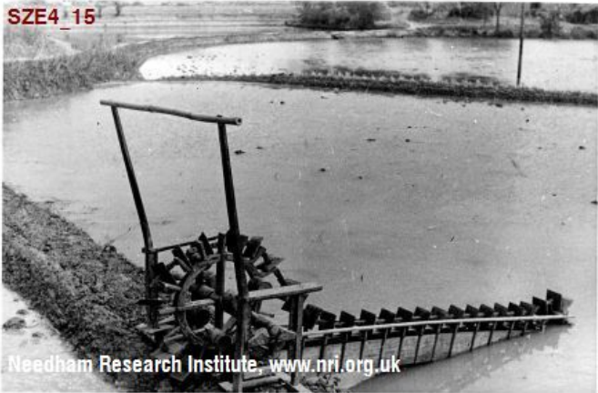
Figure 7. A dragon's backbone pump in Sichuan, China 1943. Photo by Joseph Needham.
