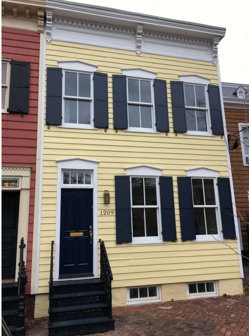
Figure 21: The exterior of 1209 Prince Street in 2020. The siding, windows, front door and transom, shutters, and front steps and railings have been re-replaced to better reflect the home's original style. The only visible exterior building elements that were not removed in the ongoing renovation are the brick foundation and the modillion—everything in between has been replaced once more. As the siding most likely consists of new growth wood and the windows are modern simulated divided light units with a limited warranty, they will probably be fully replaced once again in another thirty years' time. Photo by author.
