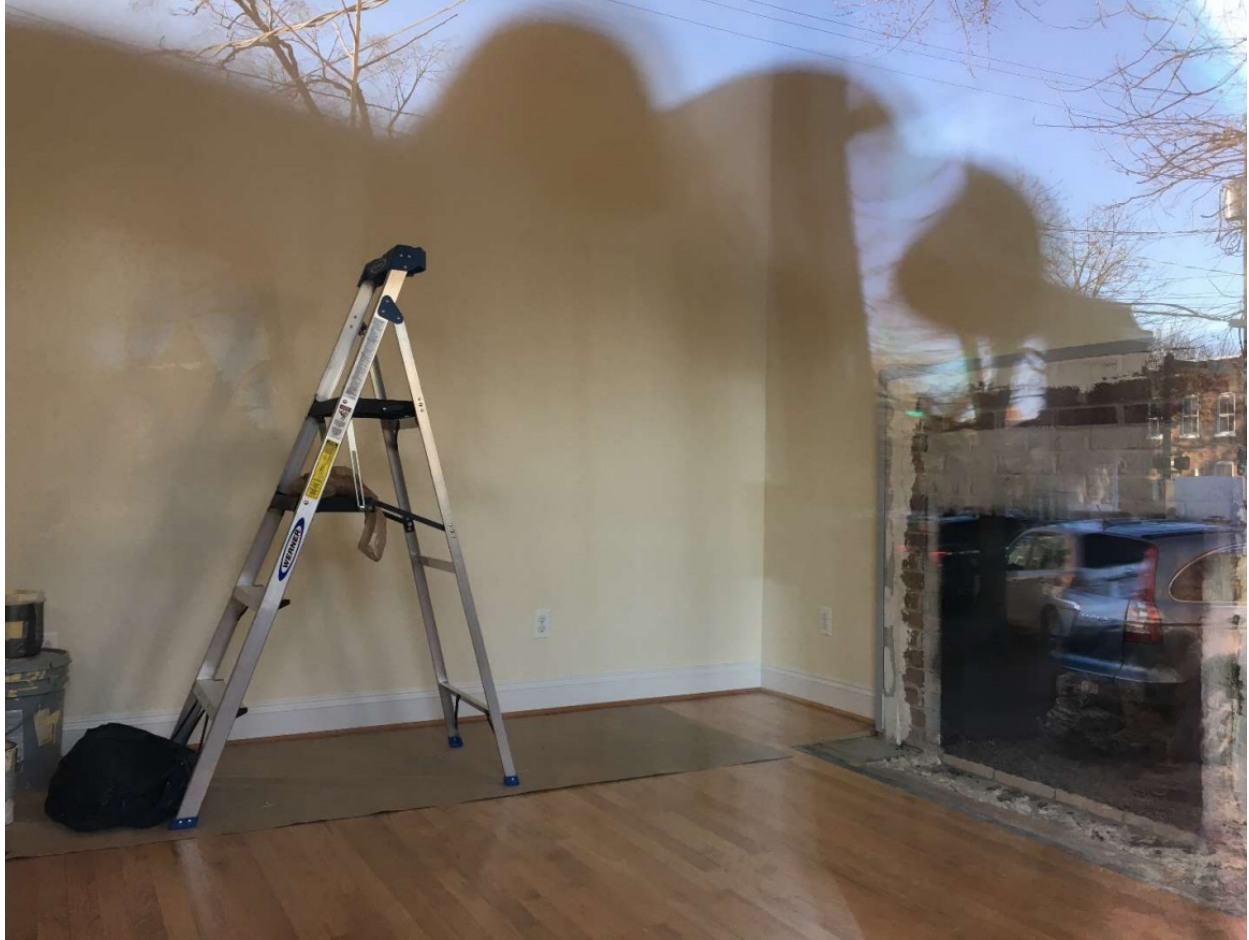
Figure 22: In 2017, one could look from the sidewalk straight through the interior of this house to the backyard. As is visible in this 2020 photo of the interior space at 1209 Prince Street, the floors, baseboards, and wall plaster have been fully replaced. Some or all of the wall framing behind that plaster may have been replaced as well. The fireplace surround has been removed and will likely be replaced soon. The floors clearly differ from those installed in the 1980s in color and grain, and the baseboards appear taller than those in earlier photos reflecting the 1980s renovation. Is the house due to be fully gutted once again in another thirty-five years? Photo by author.
