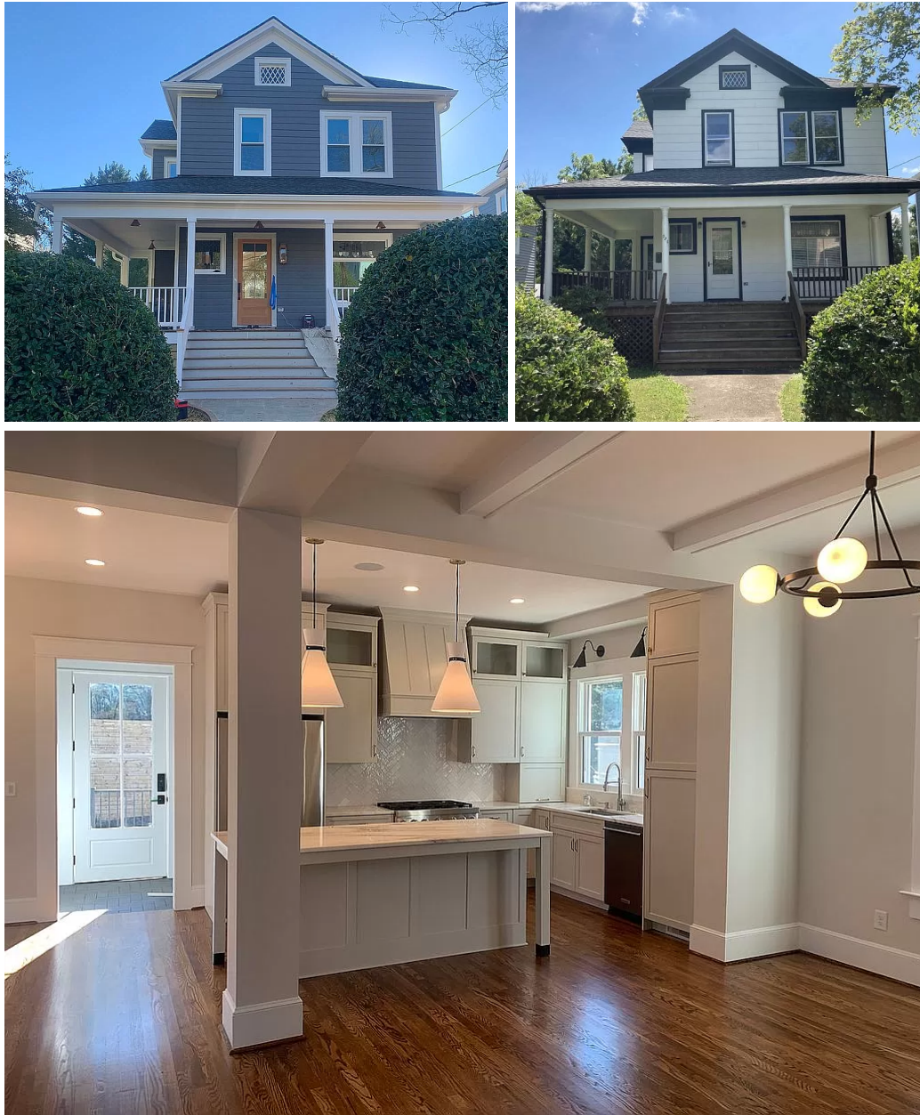
Figures 44-46: This home on Lexington Avenue was preserved only nominally in the last several years when it was gutted, re-clad, and saw its historic windows replaced. It is difficult to know just how original the interior would have been before its recent renovation, but the exterior has gone from largely original (wood siding often remains under asbestos cladding seen at top left) to an exterior whose design has not been altered, but is largely clad in modern materials of vinyl or fiberglass windows and fiber cement siding. 133 No new shade trees appear to have been planted as part of this project.
