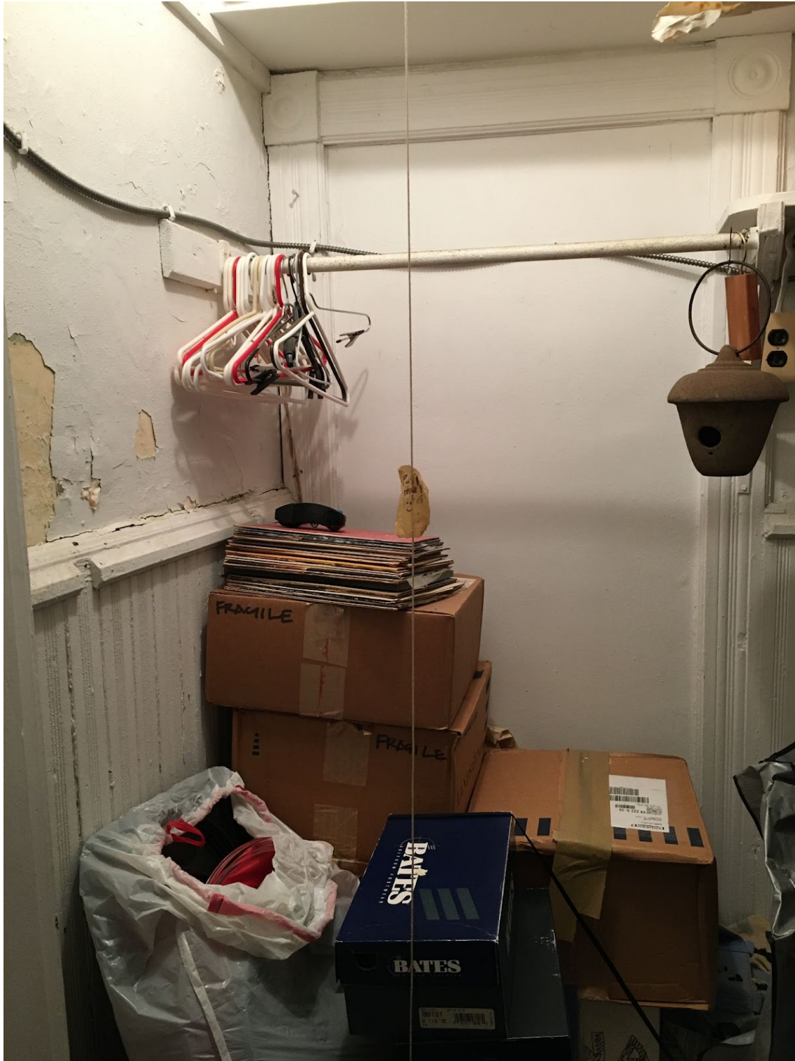
Figure 30: Door II as seen from Door I. Original surrounds indicate the location of a former doorway that has been filled in. Original beadboard on all four inside walls of the closet mark this layout as original as well. Photo by author.
