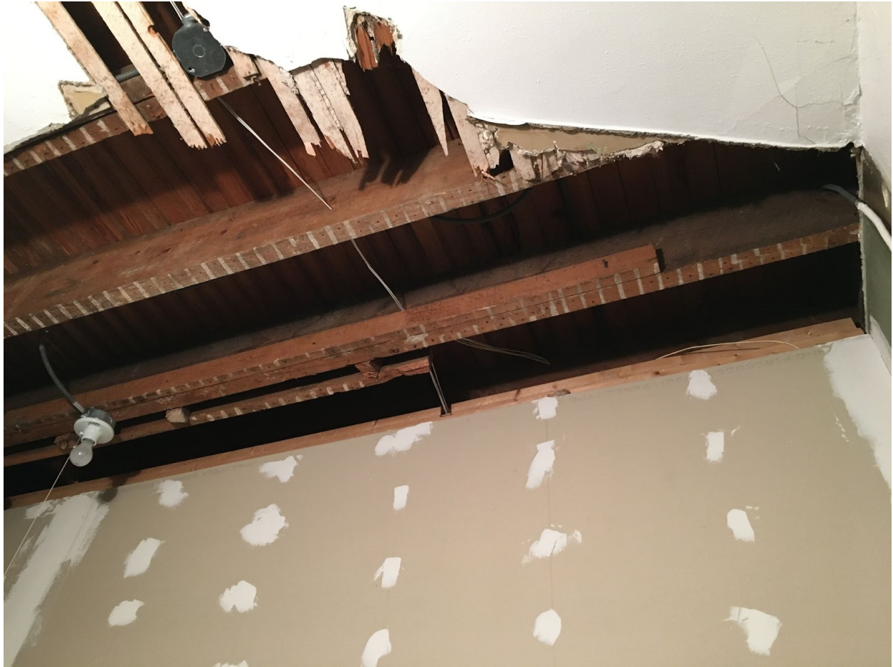
Figure 32: Note the evidence of former wall framing just to the right of the light fixture above. When the plaster was removed to move this original wall in 2002, the location of a former doorway was indicated by the absence of wall framing in the shape of a door just to the right of the remaining studs, labeled on the plan as doorway III. Photo by author.
