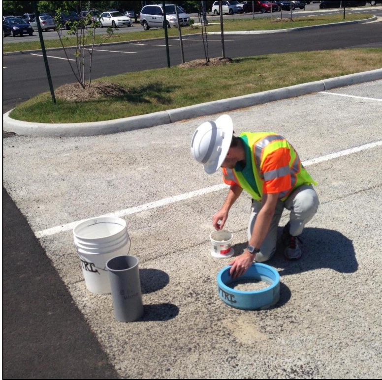
Figure 1: Stringfellow Park and Ride checkup 6 months after placement using ASTM C1701 for infiltration rate
