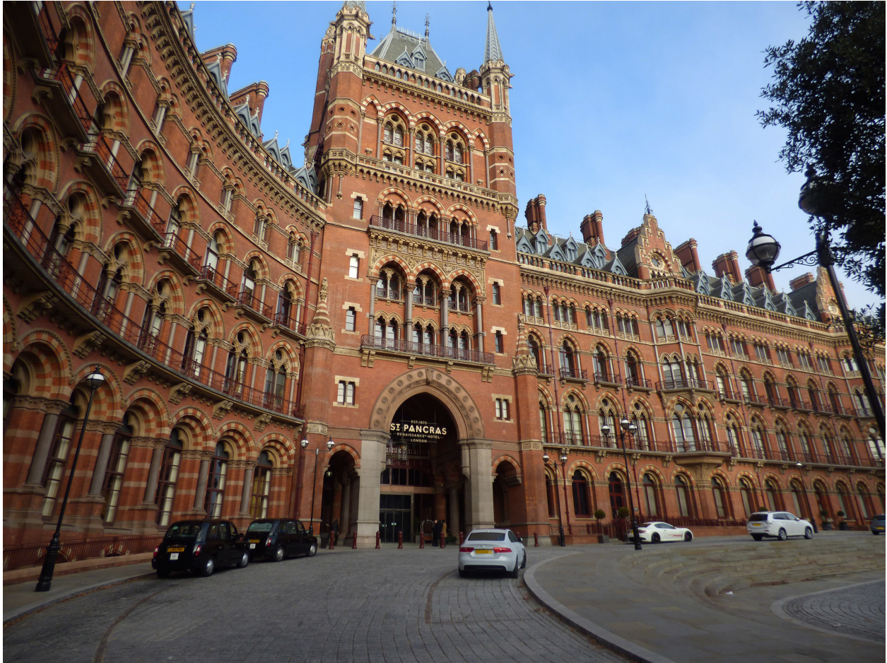
Figure 21: Midland Grand Hotel, St. Pancras, London. George Gilbert Scott, 1870s. Hotel is part of St Pancras rail station next door. A combination of medieval Gothic appearance with a modern, industrialized function.
