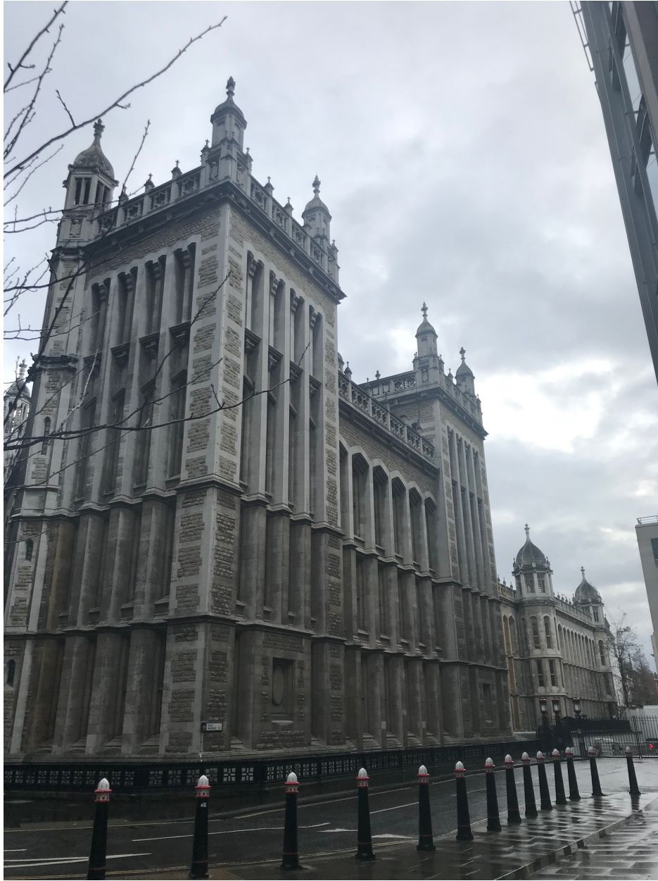
Figure 20: Former Public Record Office, Chancery Lane (viewed from New Fetter Street), London. (Maughan Library). James Pennethorne, 1850s.
