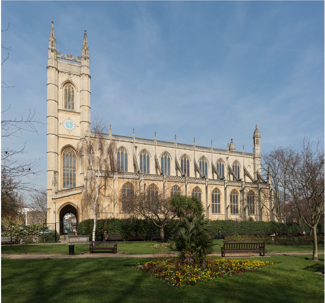
Figure 6: St. Luke's Church, Chelsea. James Savage, 1824. One of the Gothic "Waterloo Churches" from the 1818 First Church Building Act.
