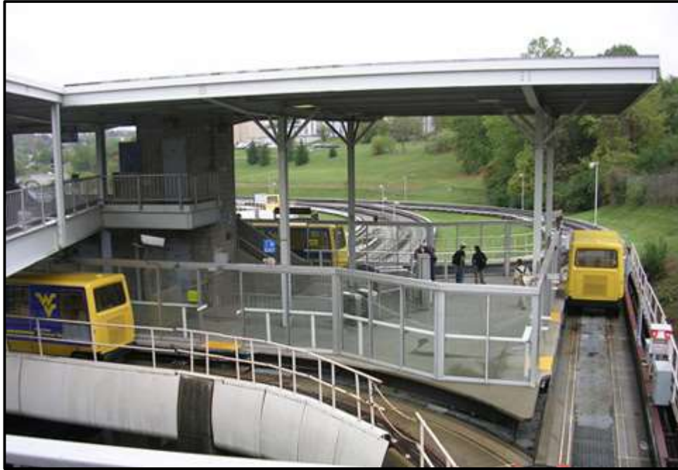
Figure 2: PRT Station Here is the PRT Engineering NB station at WVU. Cars can stop at the station or continue around the station if the destination is a different station. This station was recently closed indefinitely due to a rock fall (Rail System, 2015).
