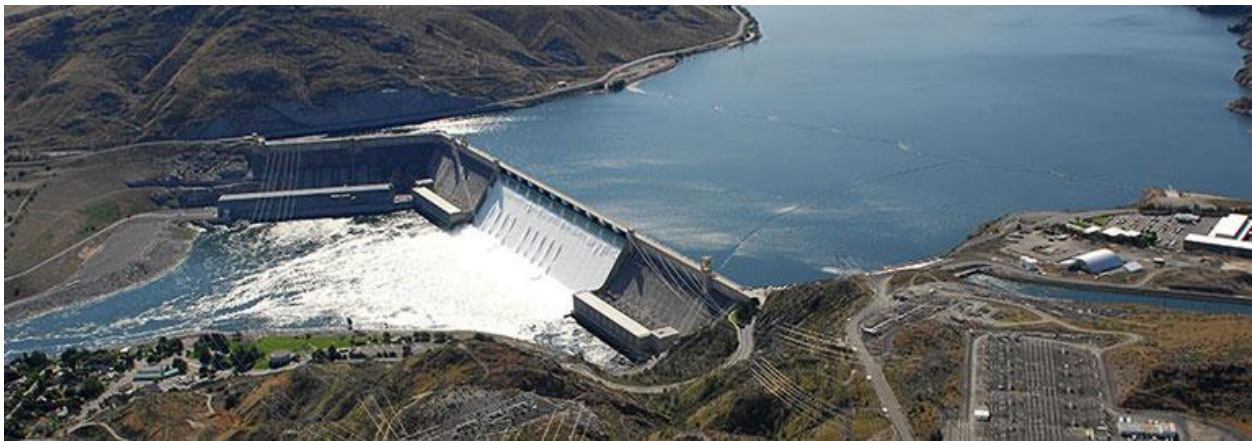
Figure 2. The Grand Coulee Dam, as shown by the USBR (2023).
