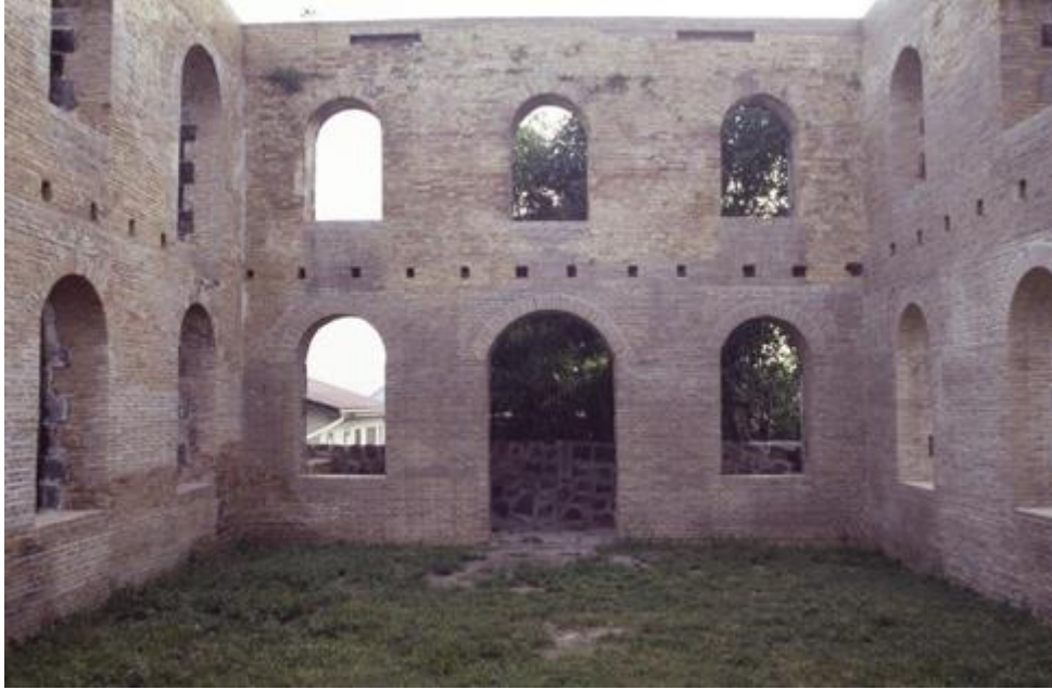
Image 5.11: Honen Dalim Synagogue ruins. Interior view, showing the west entrance and remnants of gallery supports. Photo credit: Louis Nelson, 2010; accessed on Artstor; all rights reserved by creator
