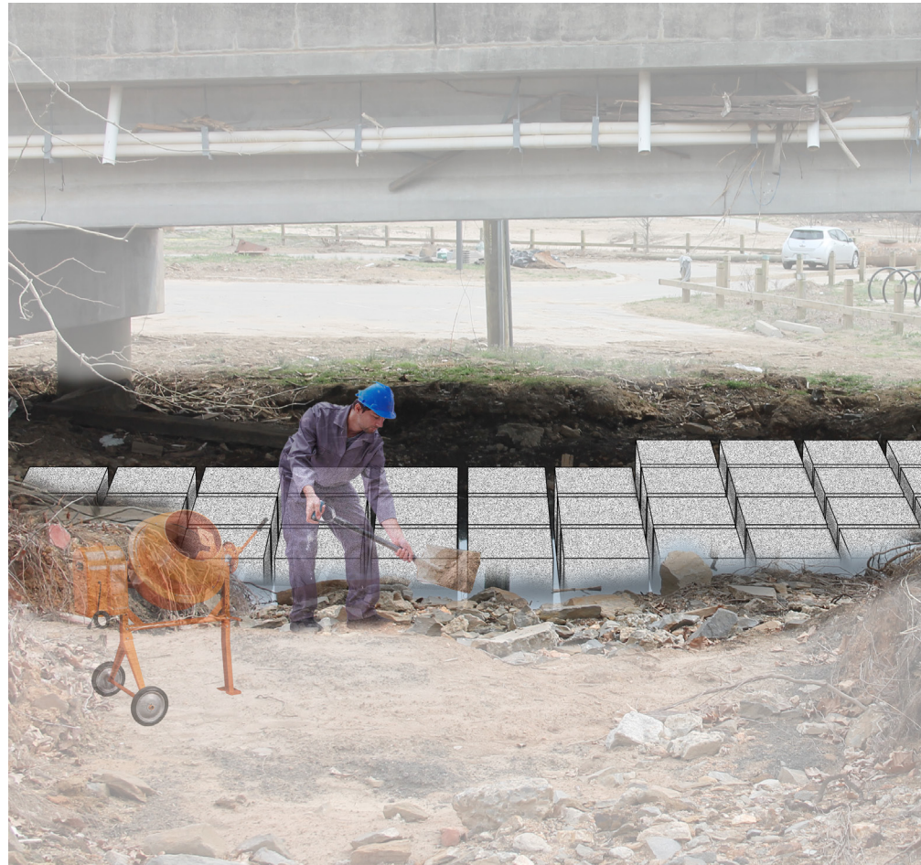
Bridge Stability is at structural risk with washout and erosion from flooding events. The creation of a permeable plane of energy dissipators, like large concrete blocks, can break up water fast while acting as a platform for walking.
