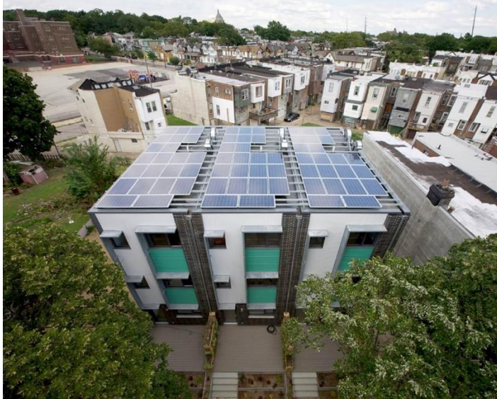
Figure 2. Belfield Townhomes' Rooftop PV System (Source: Onion Flats Architecture, n.d.)
