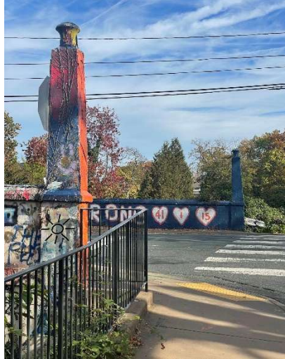
Fig. 3.2.2. Beta Bridge at UVA, column view
