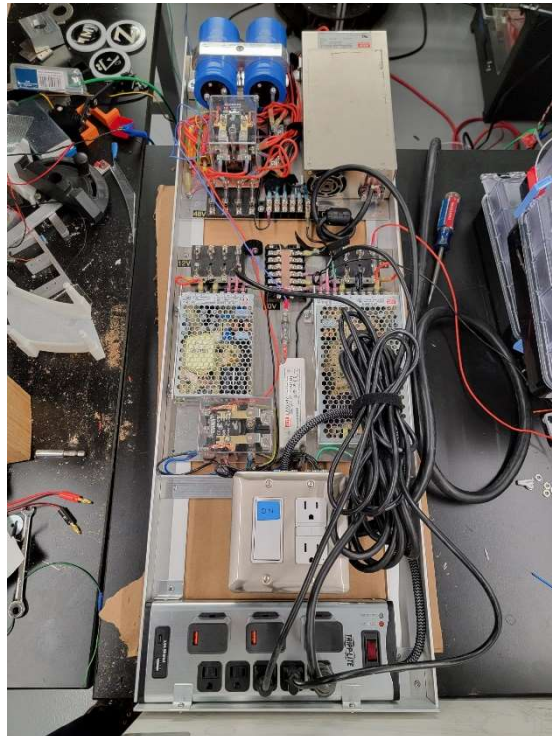
Fig. 4.5.2. Finished and mounted power supply for the pinball machine
