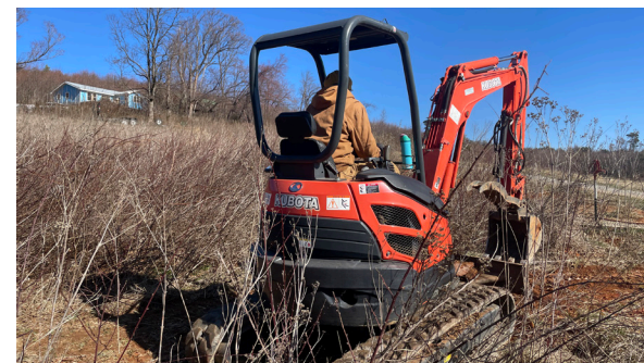
Digging berms and basins with excavator
