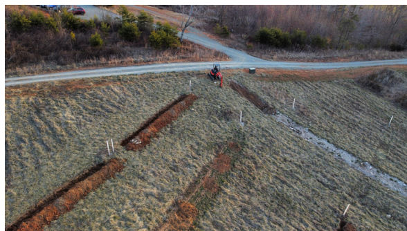
Tree planting with excavator
