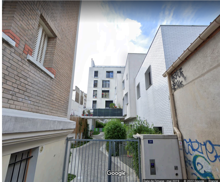
Figure 3.11: 31 rue Ramponeau, May 2019
