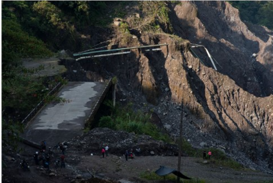
Figure 6. Devastating effects of erosion. The picture above displays the destruction wrought by the 2020 disaster, where erosion caused the sliding and collapse of a highway, portion of a town, and utility lines. (Dube & Steinhauser, 2023).
