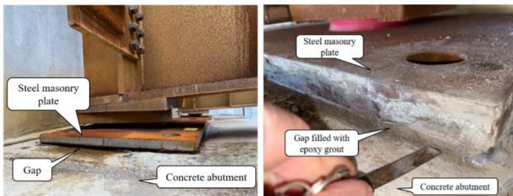
Figure 2. An example of a gap repair between a beam end and a concrete abutment (Provines, 2022).
