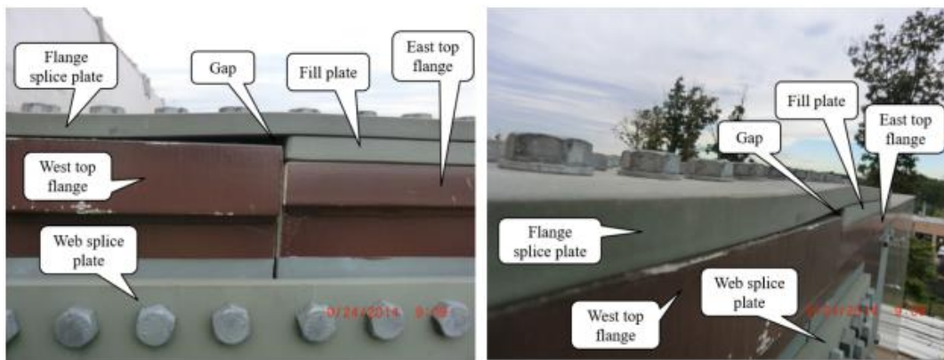
Figure 1. An example of a gap repair between a flange on a bridge (Provines, 2022).
