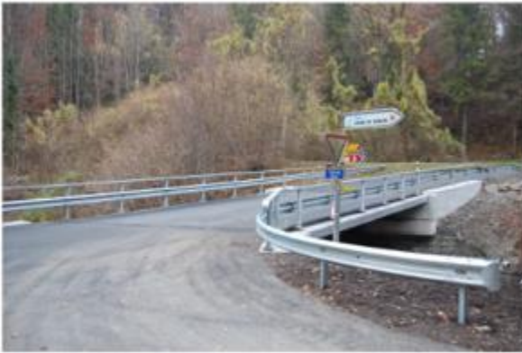
Figure 11. New Avançon bridge, Bex, Switzerland; with the installation of the semi-integral bridge comprising GFRP deck bonded onto steel, longitudinal girders, and supported by cross beams. (Keller et al., 2013)
