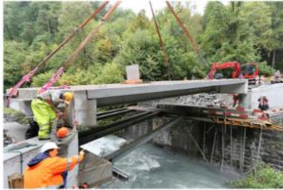
Figure 11. New Avançon bridge, Bex, Switzerland; with the installation of the semi-integral bridge comprising GFRP deck bonded onto steel, longitudinal girders, and supported by cross beams. (Keller et al., 2013)
