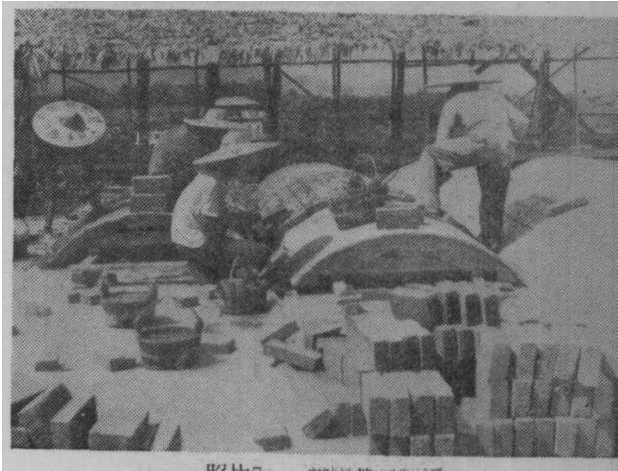
Fig.25 Installation of the Arched Roof as an Insulation Layer
