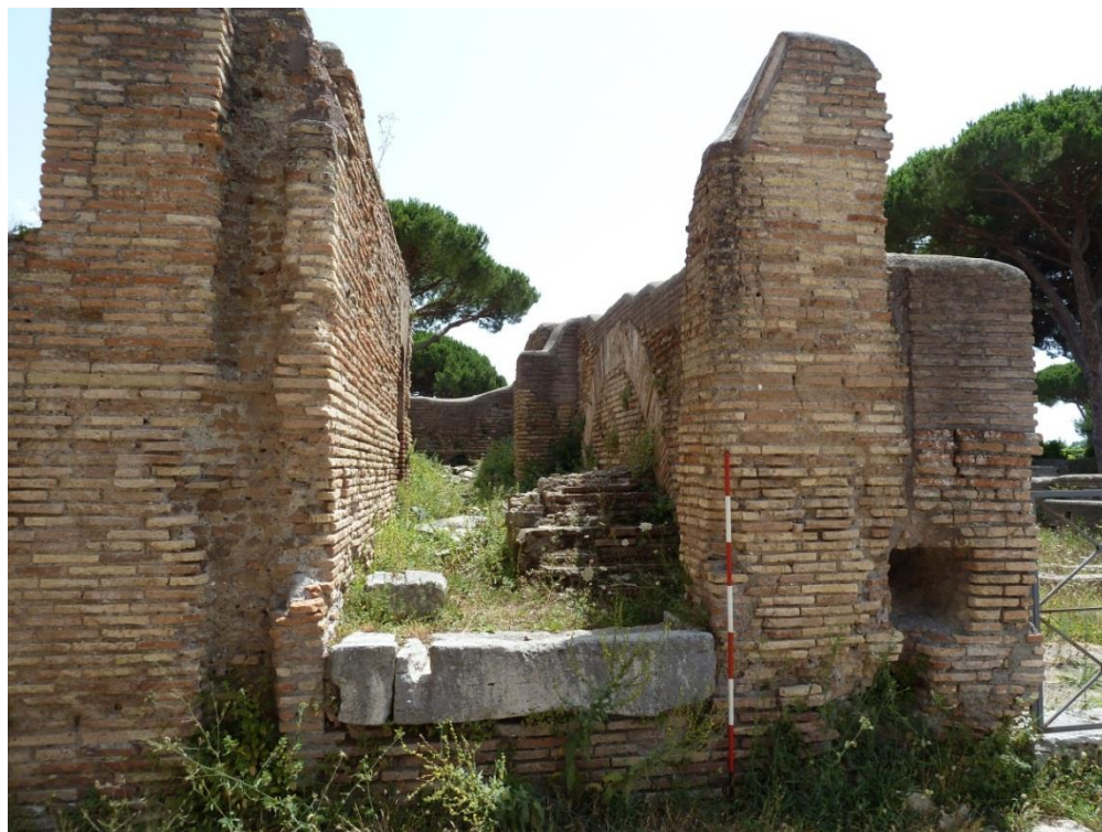
Figure 3-49: Door AE with Access to Room a2
