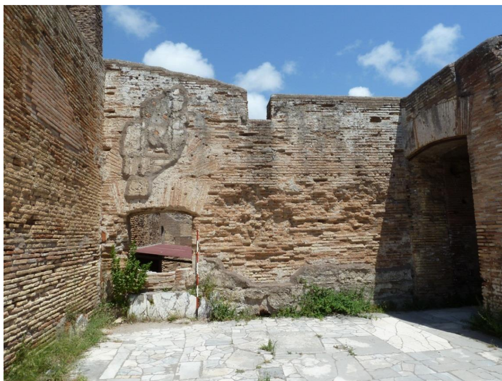
Figure 3-174: View Looking East in Room 20
