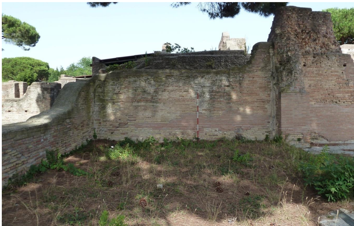
Figure 3-110: View Looking East into Room 12
