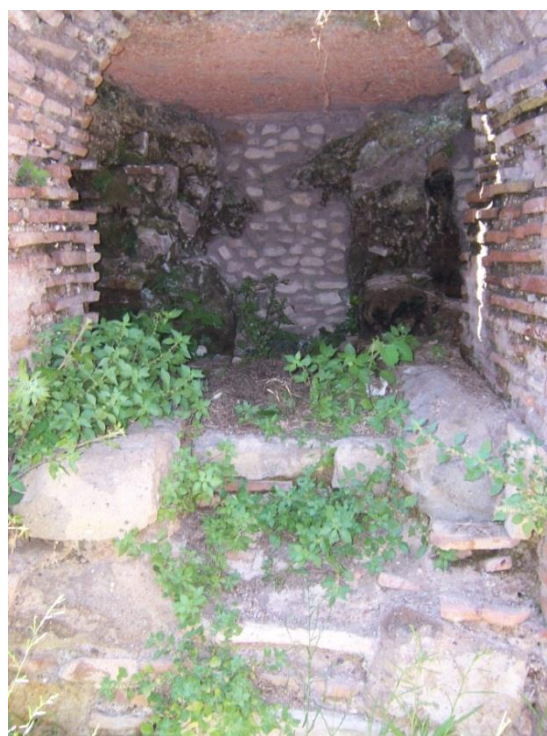
Figure 3-144: Furnace Opening for Room 17 on South Side in Substructures
