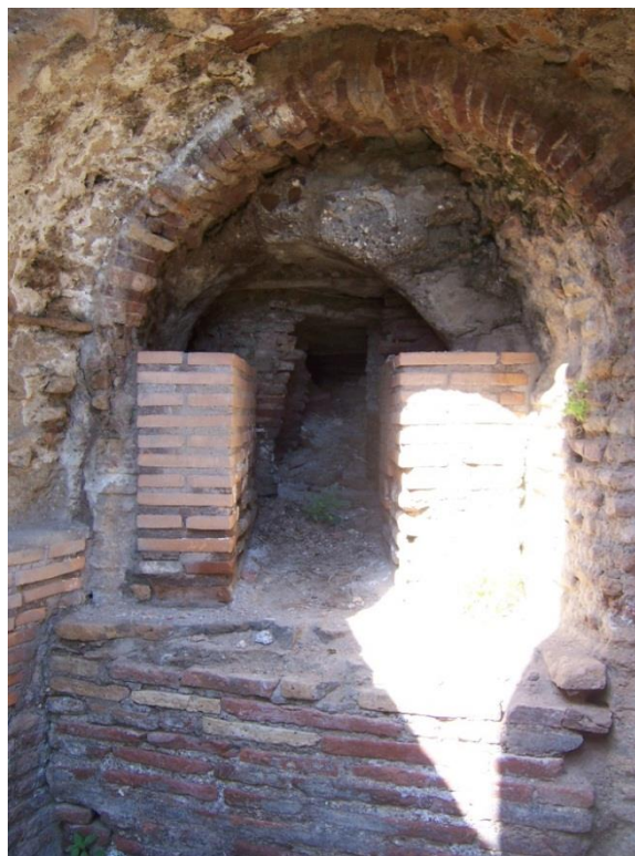
Figure 3-152: Furnace Opening for Room 18 on Southwestern Side in Substructures
