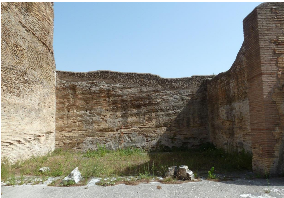
Figure 3-109: View Looking South into Room 13 from Room 11
