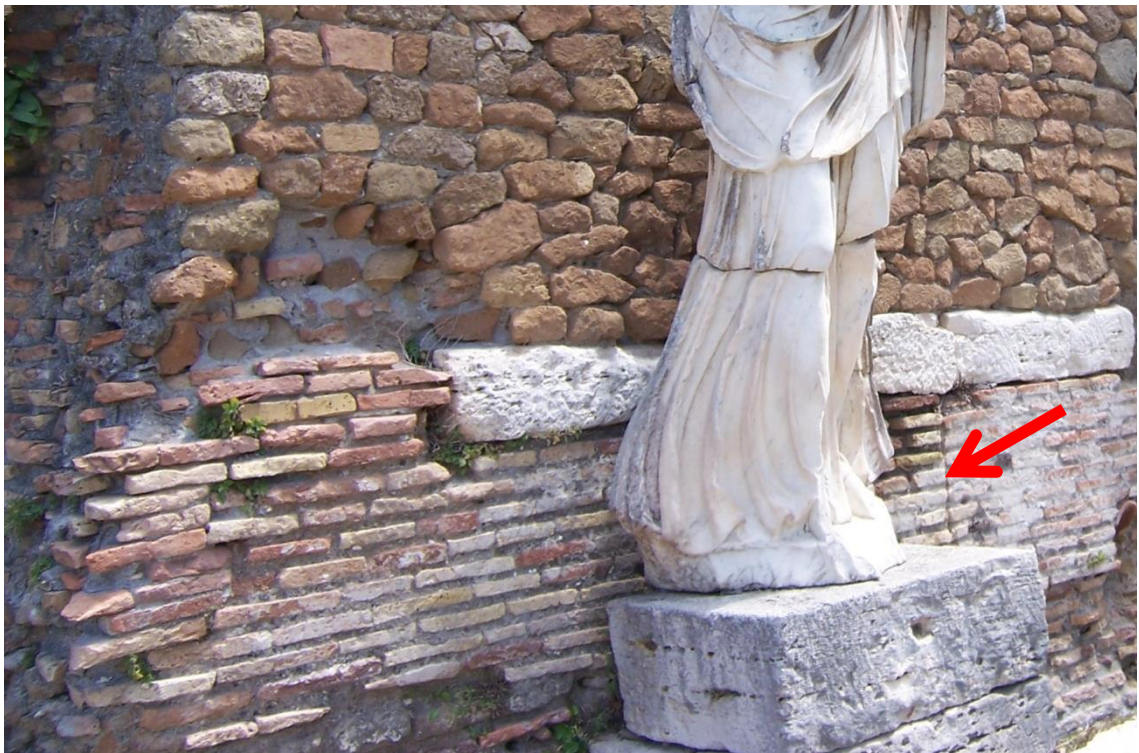
Figure 3-60: Outside of outer wall of Wall I showing Construction Seam
