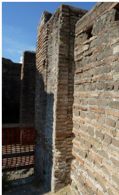
Figure 3-65: Additional Segment of Wall in Door T in Room 2
