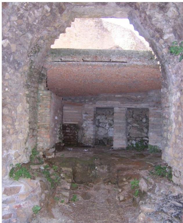
Figure 3-135: Furnace Opening with Visible Hypocaust Pillars for Room 16 in Substructures
