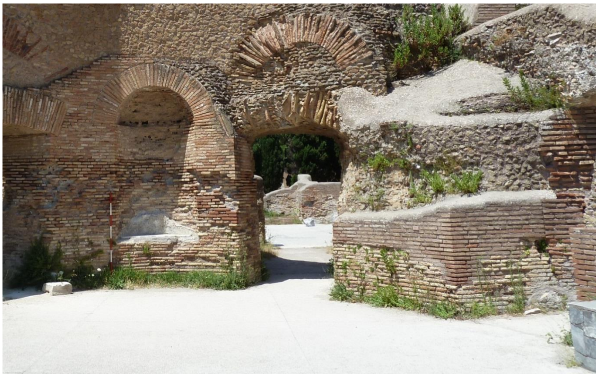
Figure 4-4: View Looking North in Room 16 showing Niche, Wall a and Wall b
