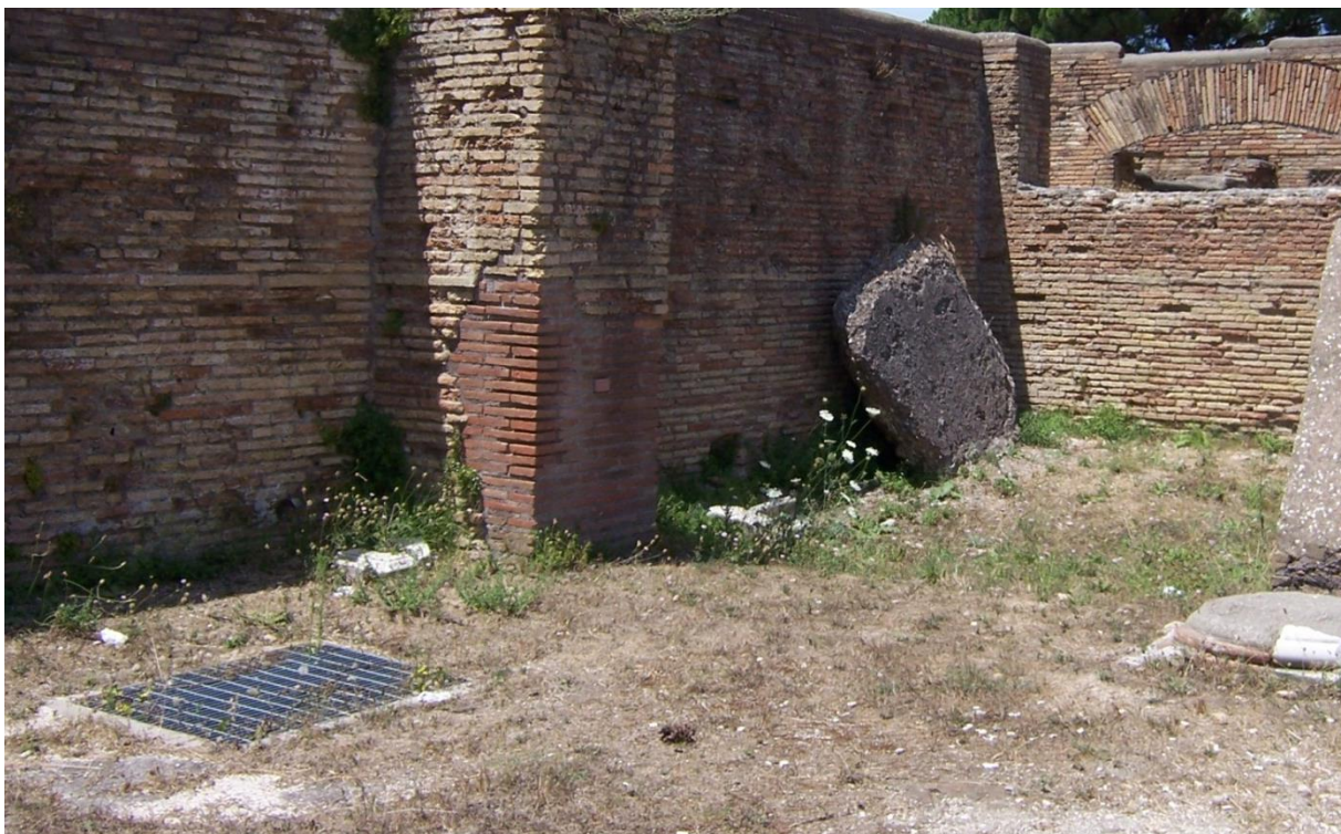
Figure 3-69: Large Drain D9 in Room 2 looking Northwest
