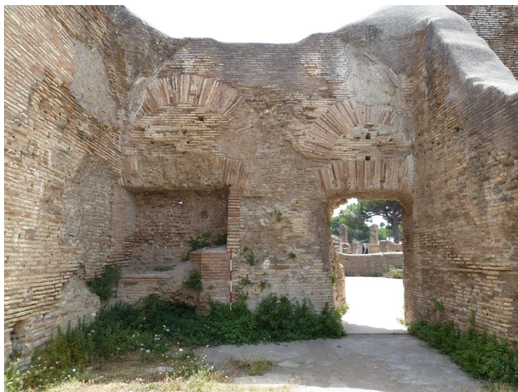
Figure 3-96: View Looking South into Room 9
