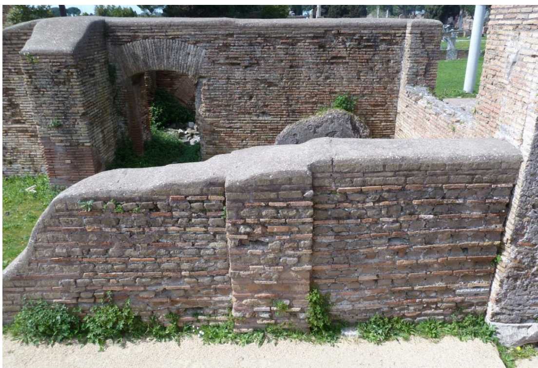
Figure 3-66: Walls z, ad, and ah in Room 2
