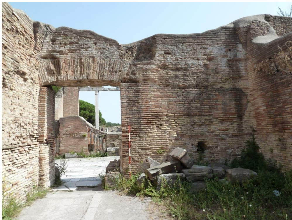
Figure 3-97: View Looking South into Room 10
