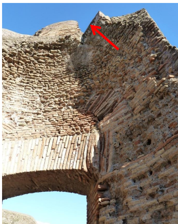
Figure 3-132: View Looking Southeast at Opening in Ceiling in Room C
