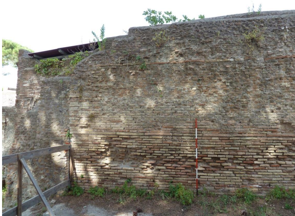
Figure 3-122: View Looking East in Room 14b towards the Caseggiato della Cisterna
