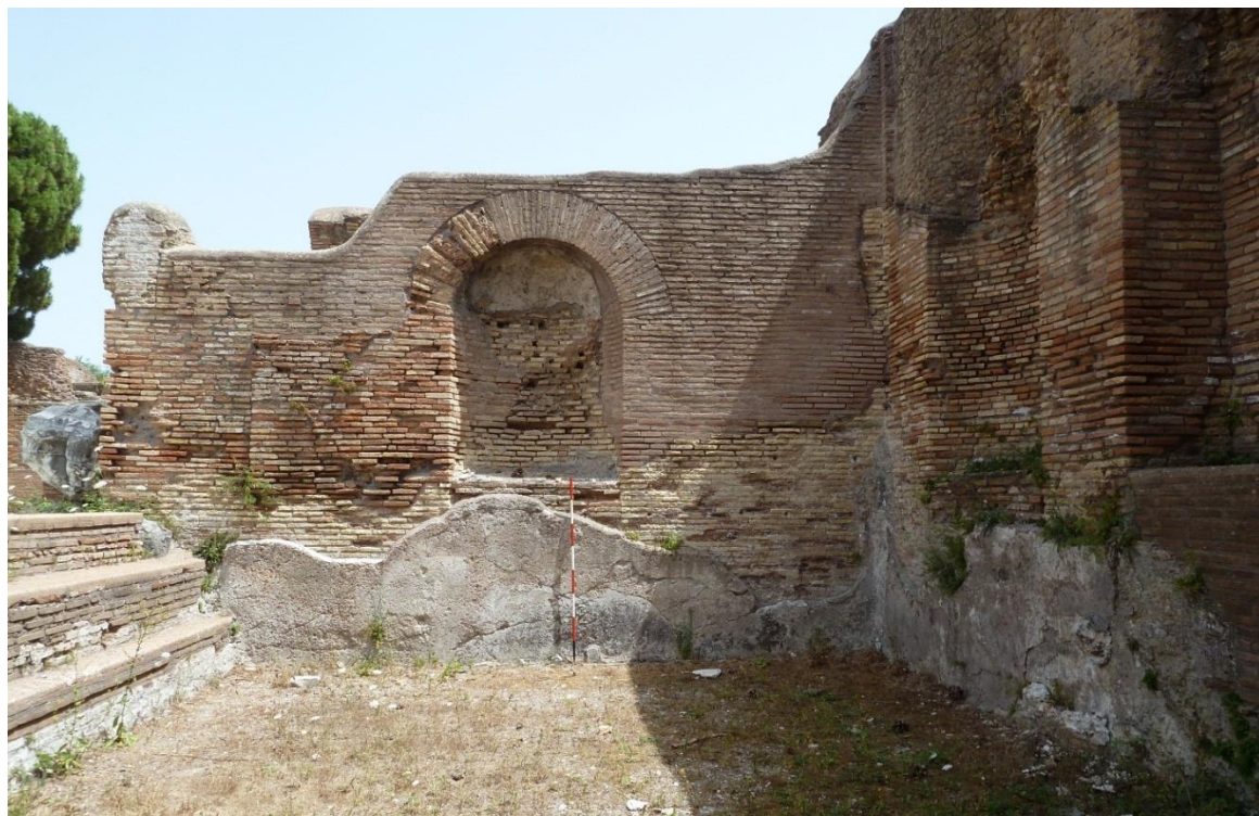
Figure 3-90: View Looking East in Pool ε in Room 6
