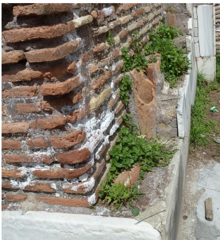
Figure 4-8: Wall Layers in Room 17
