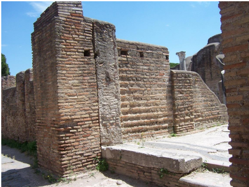
Figure 3-20: Fourth Century AD Entrance (Door T) to the Terme del Foro, Ostia
