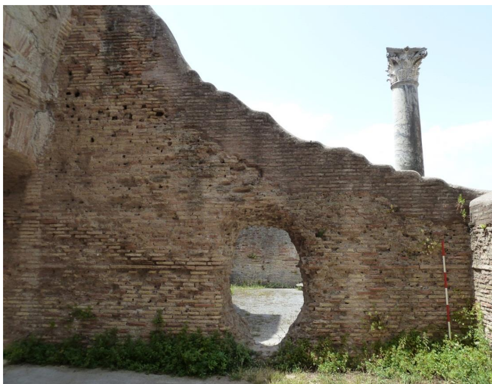
Figure 3-104: View Looking West in Room 9
