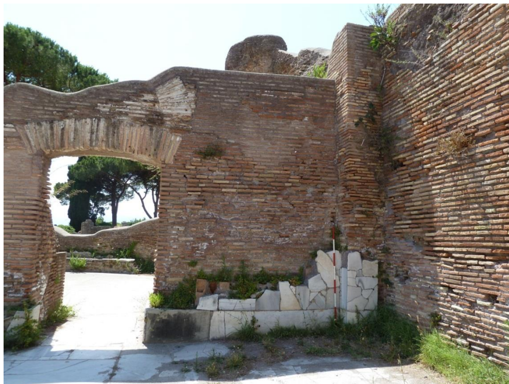
Figure 3-11: View Looking West in Room 17 showing Fortifying Pilaster and Door F
