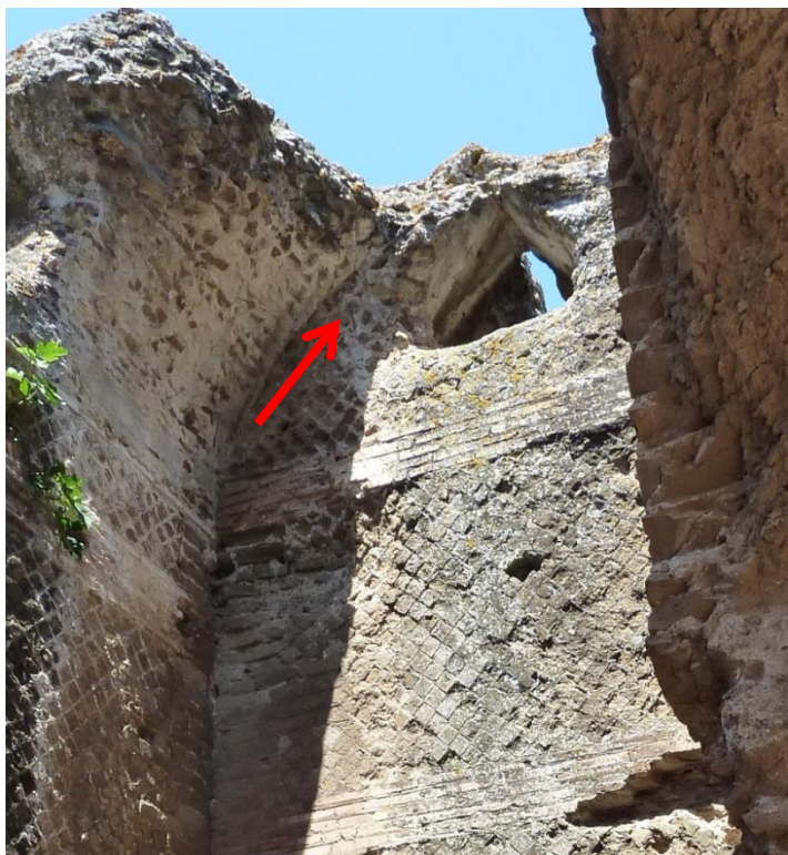
Figure 2-4: Triangular “Chimney” Opening in the Grandi Terme at Hadrian’s Villa, Tivoli
