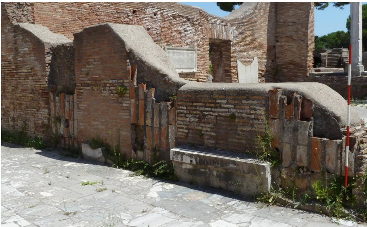
Figure 4-9: View Looking Southeast in Room 20 showing Intermittent Rows of Tubuli
