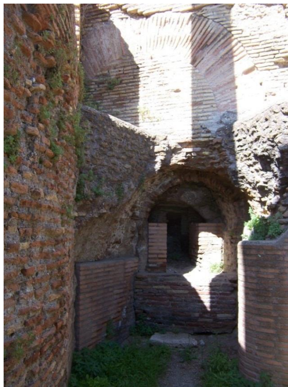
Figure 3-149: Furnace Opening for Room 18 on West Side in Substructures
