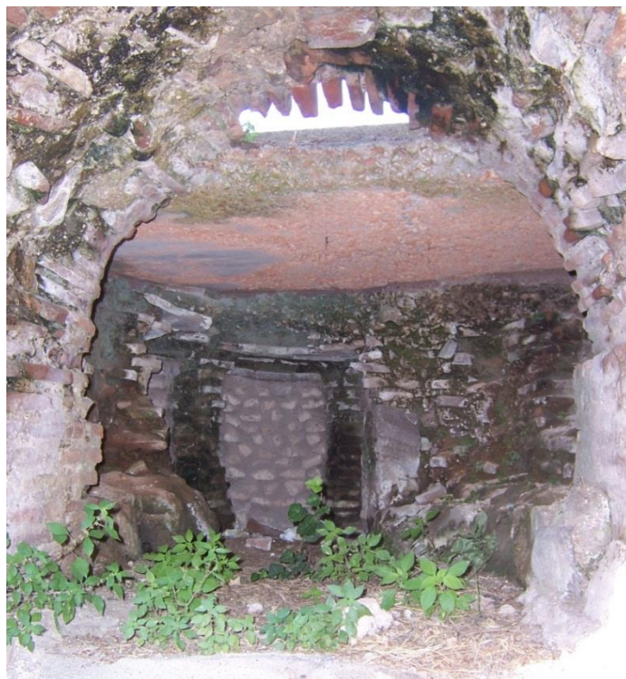
Figure 3-143: Furnace Opening for Room 17 on Southwest Side in Substructures
