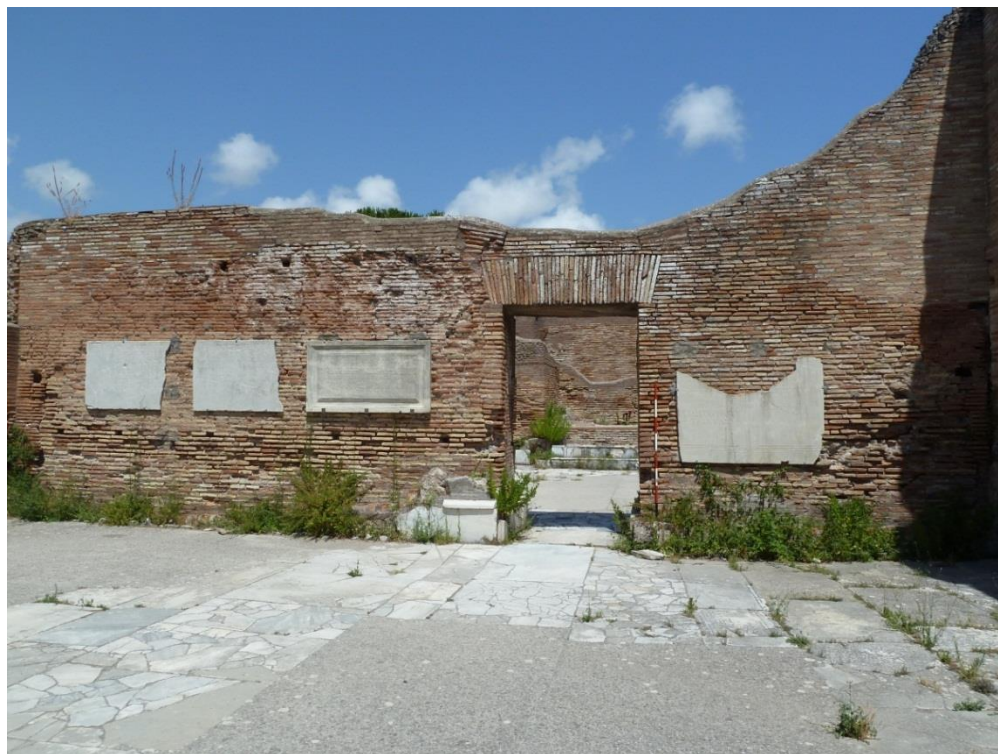
Figure 3-155: View Looking East in Room 18
