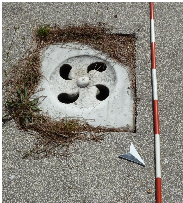
Figure 2-24: Drain D5 in the Terme del Foro, Ostia
