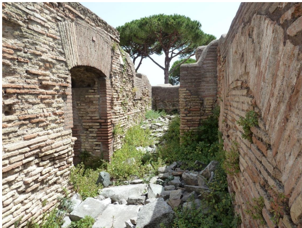
Figure 3-48: View Looking South in Room a2
