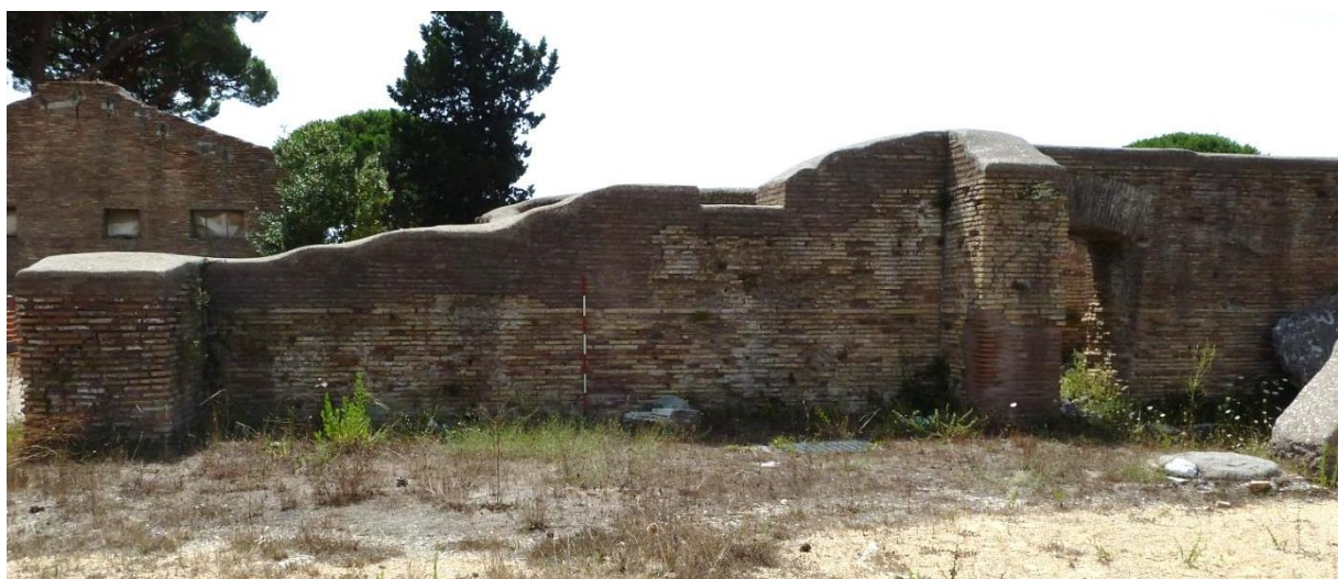
Figure 3-70: View Looking West in Room 2
