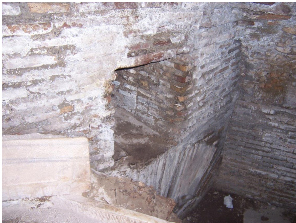
Figure 3-167: Furnace Opening for Room 19 in Southeastern Side in Substructures
