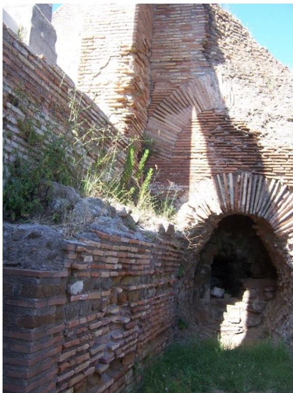
Figure 3-165: Furnace Opening for Room 19 in Southwestern Side in Substructures
