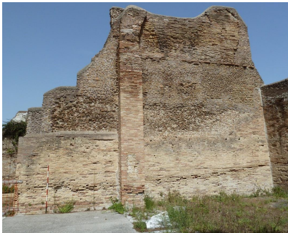
Figure 3-111: View Looking East into Room 13
