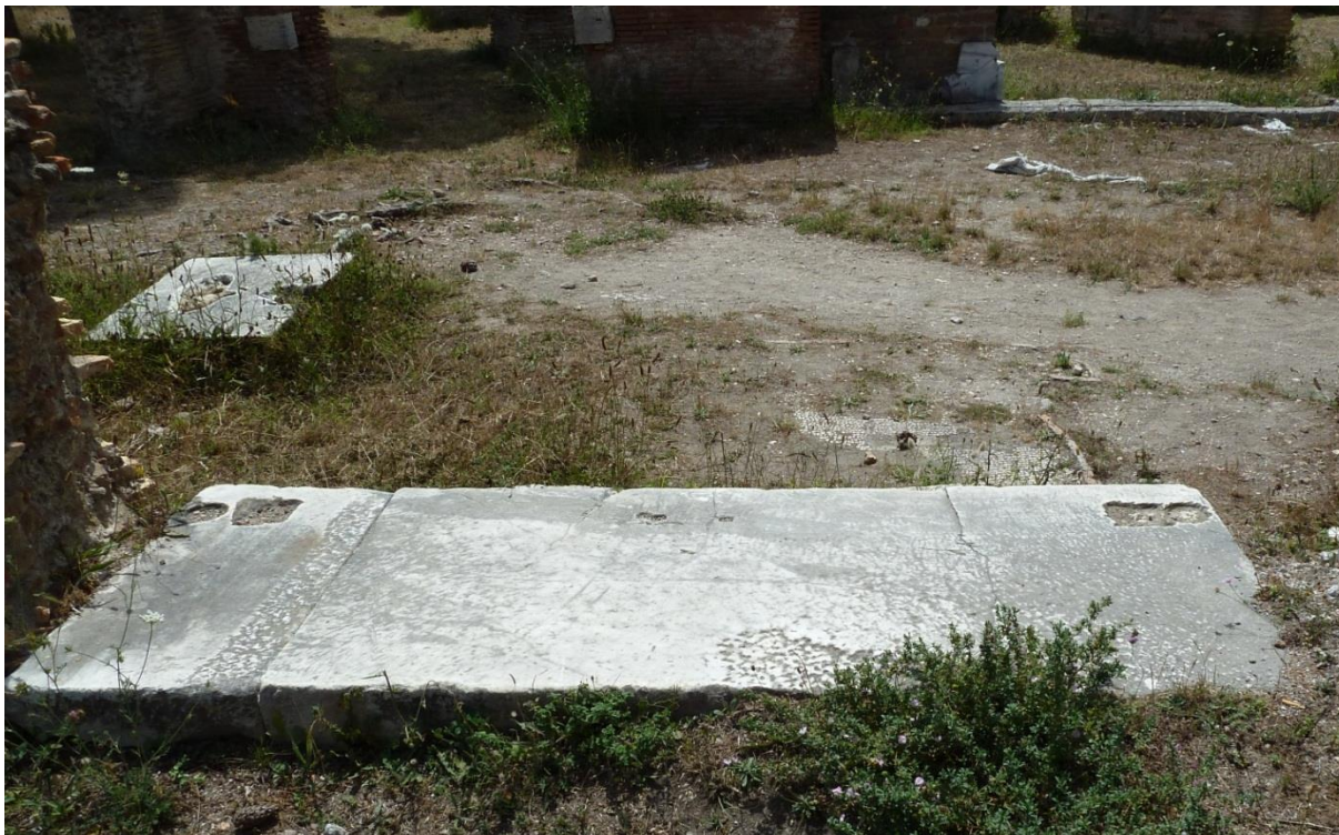
Figure 4-15: Threshold of Door AC Looking South from Room 1 to Outside of Terme del Foro
