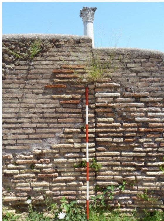
Figure 3-27: Seam in Wall of Room 16 in Terme del Foro, Ostia
