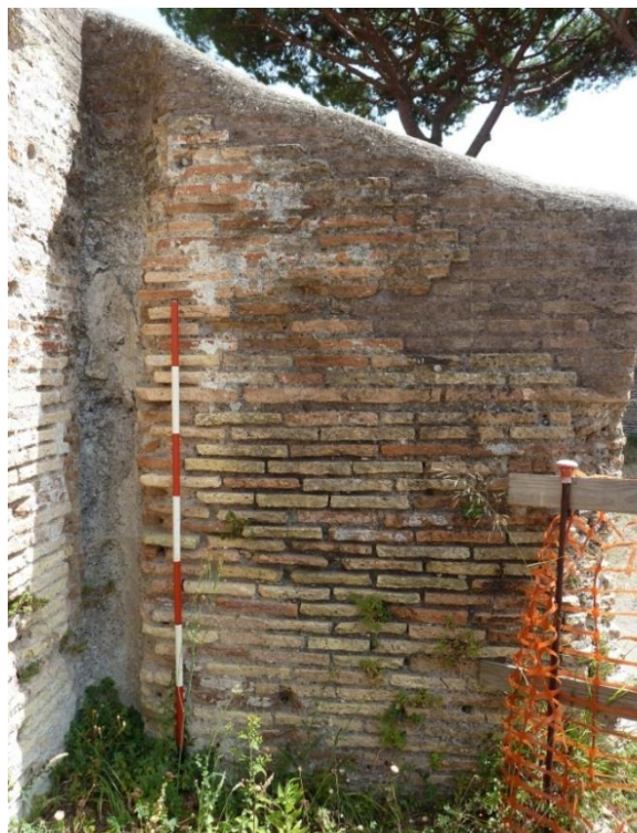
Figure 3-75: Fistulae Slot in Wall 1 in Room 2
