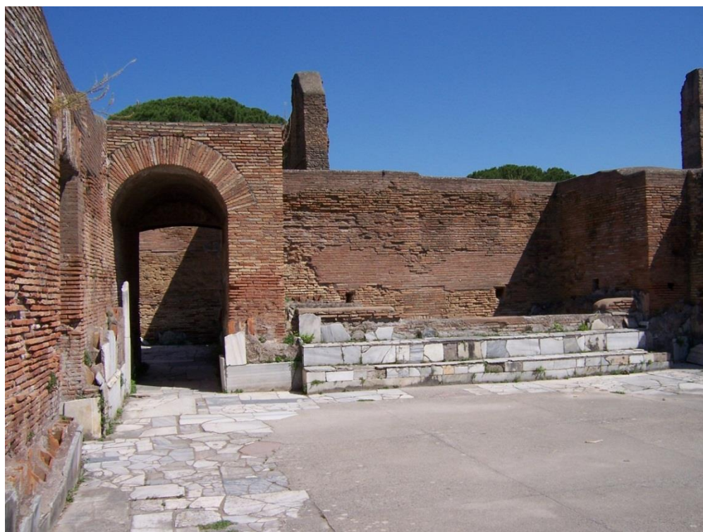
Figure 3-158: View Looking North in Room 19 showing Pool \alpha and Door K
