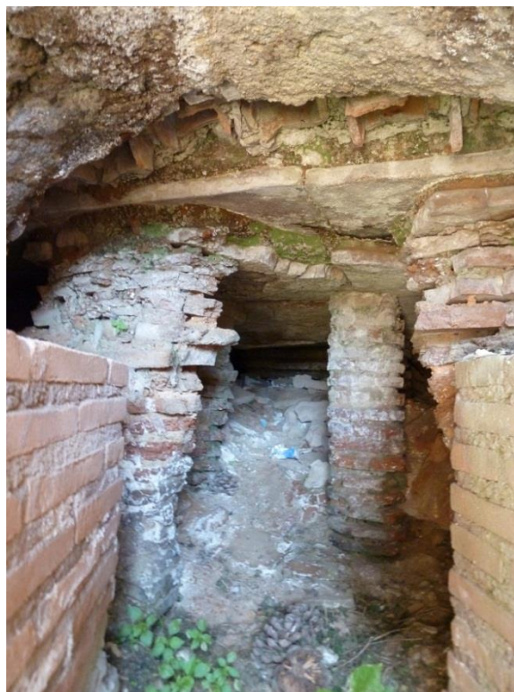
Figure 3-150: Furnace Opening showing Hypocaust for Room 18 on West Side in Substructures
