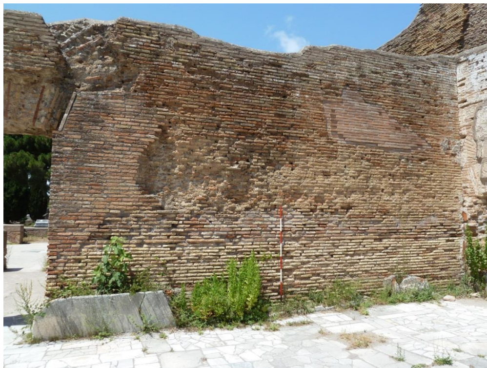
Figure 3-173: View Looking Northeast in Room 20
