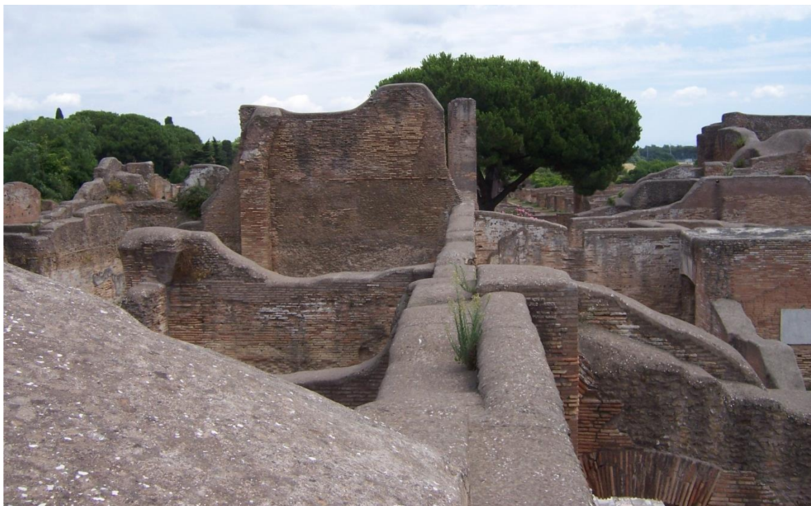
Figure 3-26: Walls Dividing Northern and Southern Sectors of the Terme del Foro, Ostia
