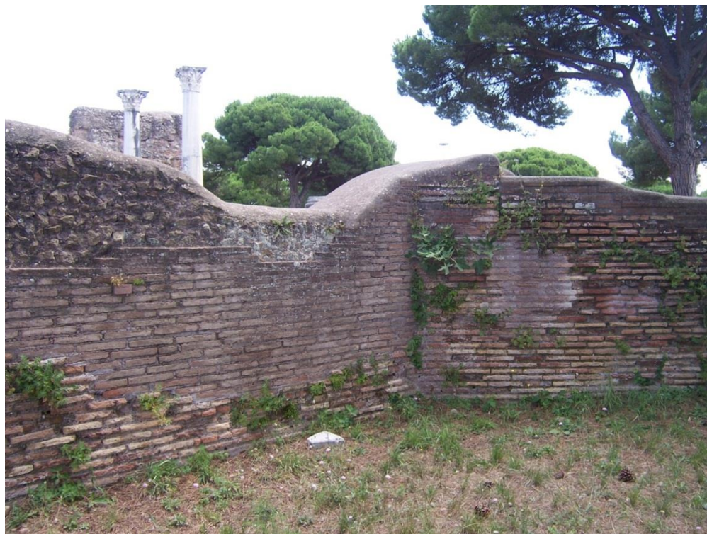
Figure 3-127: View Looking Southeast showing Window Evidence in Walls e and f in Room 15
