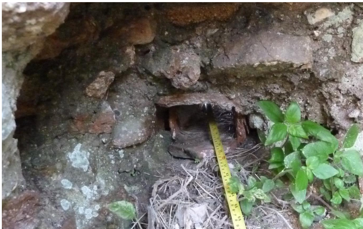
Figure 3-102: Channel between Room 9 and Rom 17
