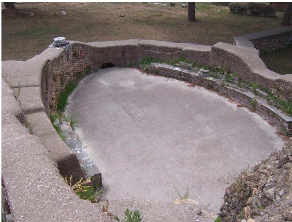
Figure 3-134: View Looking Southwest into Room 16 showing Columns C25 and C26, and Bench
