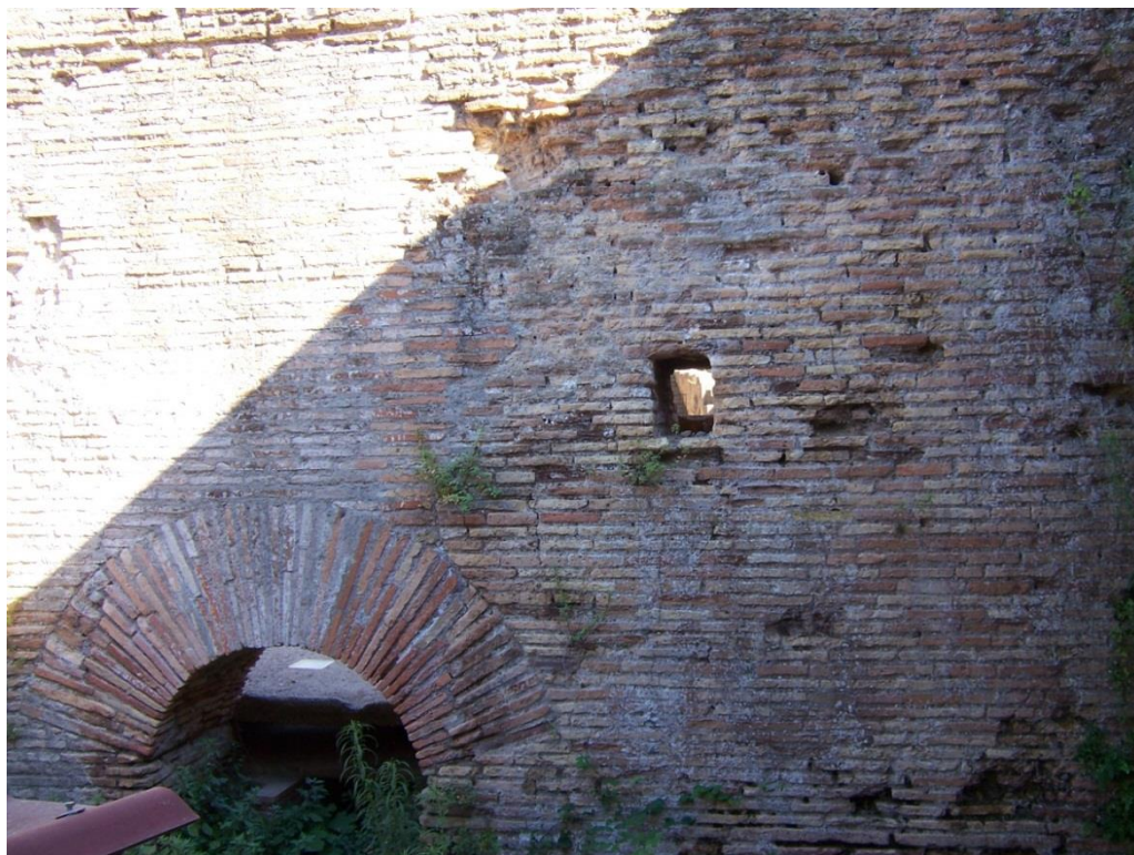
Figure 3-163: Furnace Opening for Pool \alpha in Room 19
