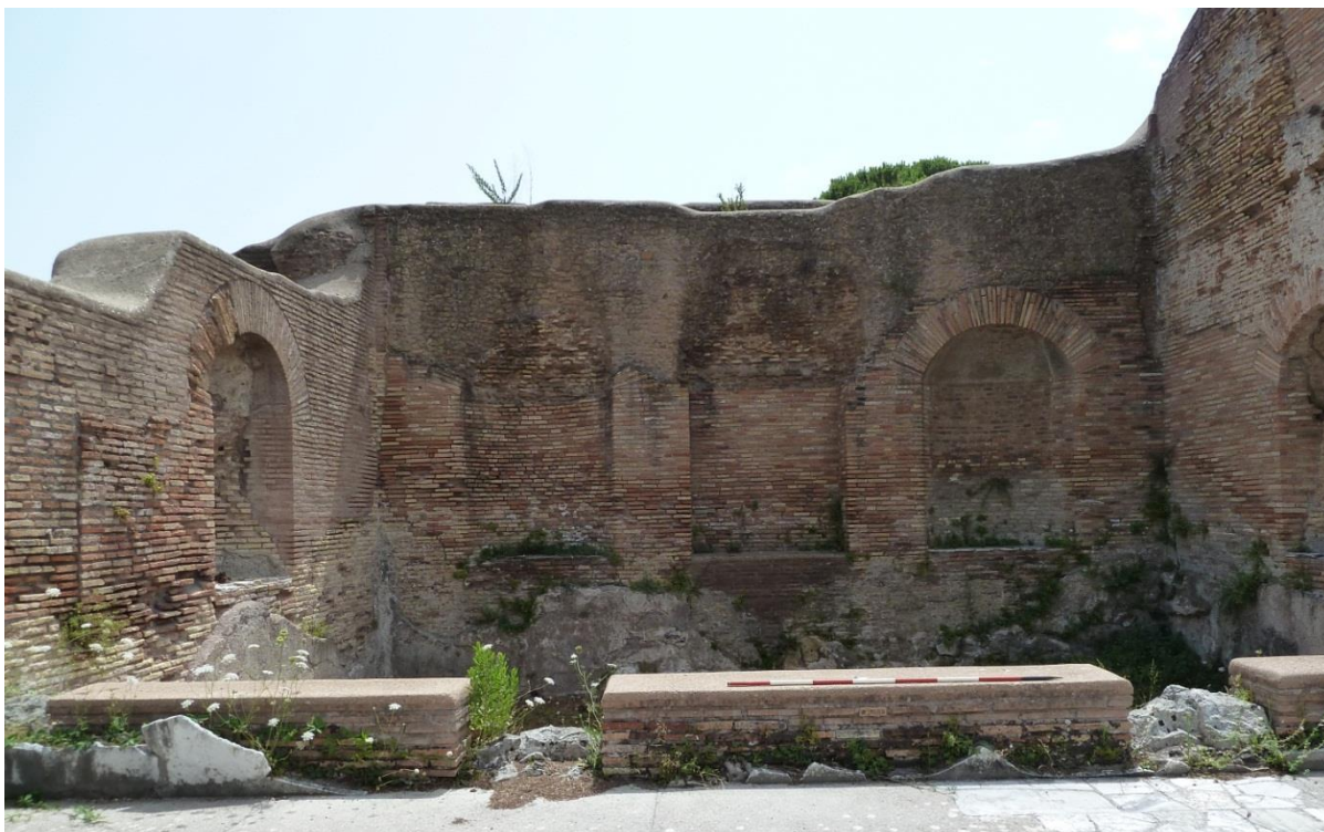
Figure 3-85: Pool ε in Room 6 looking South
