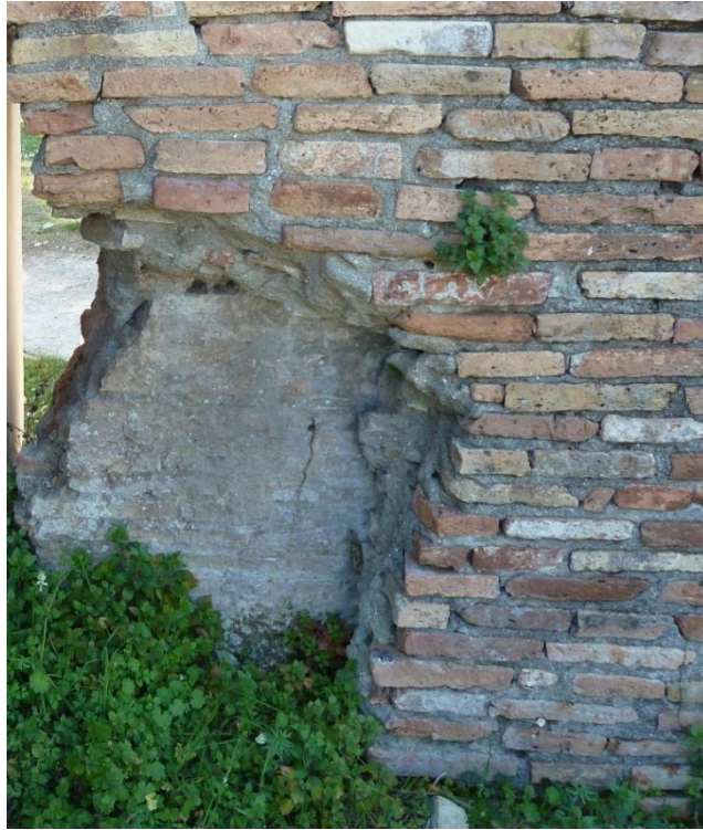
Figure 3-59: Two Walls forming Wall I in Room 1
