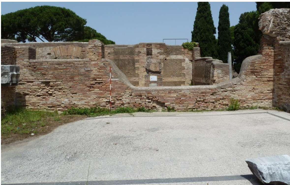
Figure 3-83: Possible Window in Room 4
