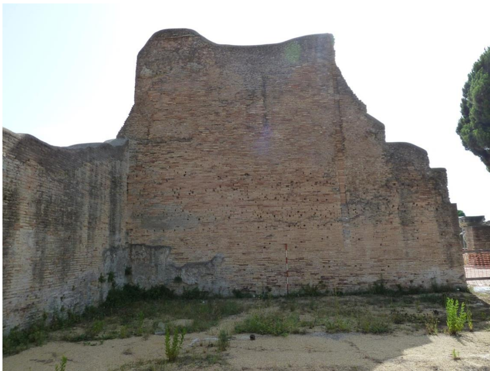
Figure 3-118: View Looking West in Room 14
