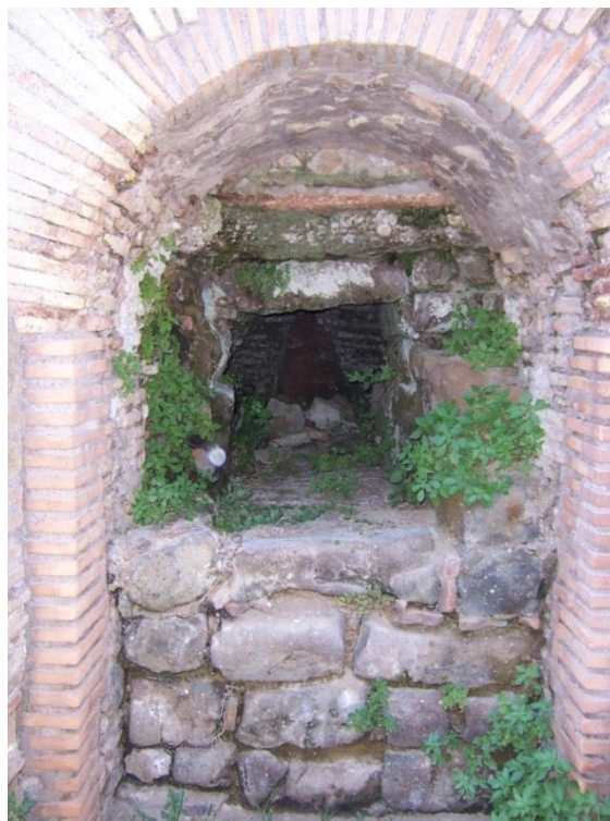
Figure 3-151: Furnace Opening for Room 18 on Central Side in Substructures
