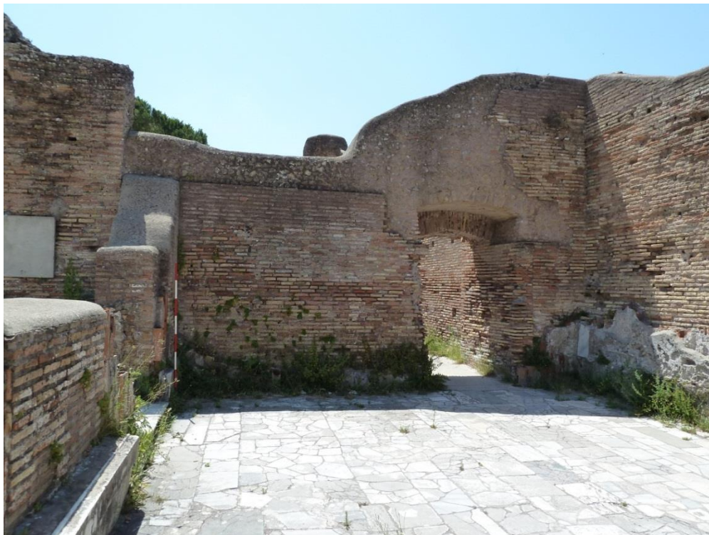
Figure 3-175: View Looking West in Room 20
