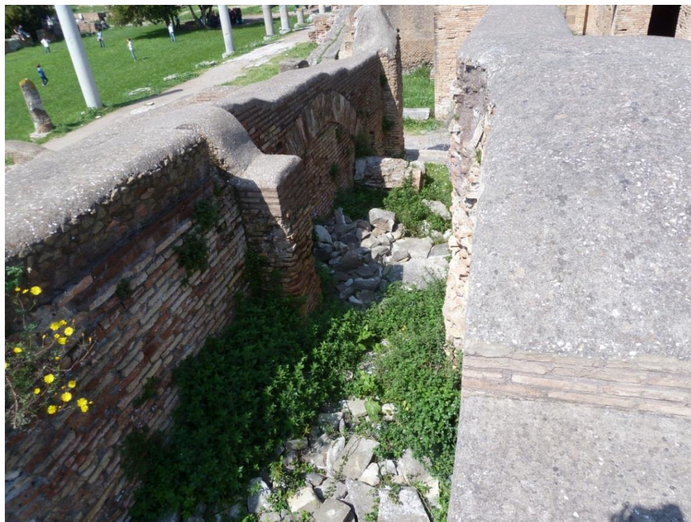
Figure 3-47: View Looking North in Room a2
