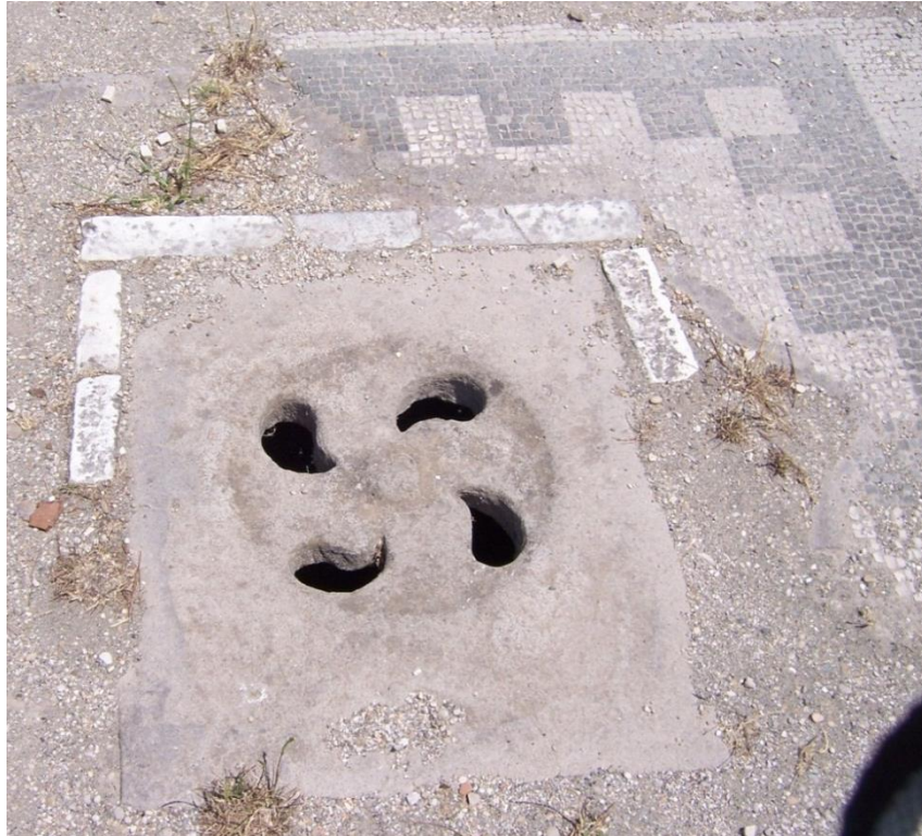
Figure 3-71: Drain D10 in Room 2
