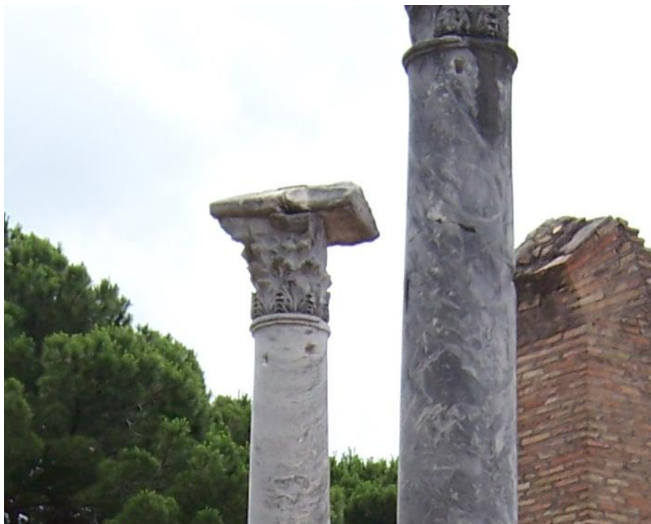
Figure 3-186: Column C30 in Room 19 showing Traces of Mortar
