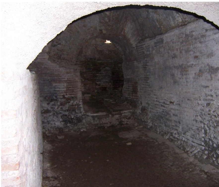
Figure 3-34: Covered Chamber near Room 19 in the Substructures of the Terme del Foro
