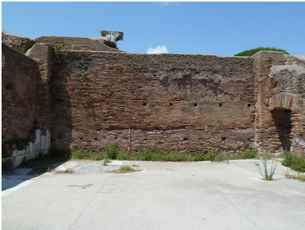
Figure 3-141: View Looking North in Room 17 showing Wall a and Door G
