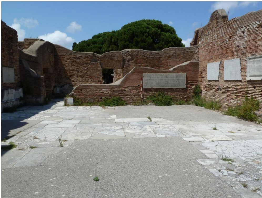
Figure 3-147: View Looking North in Room 18 and showing Door J and Walls a and b
