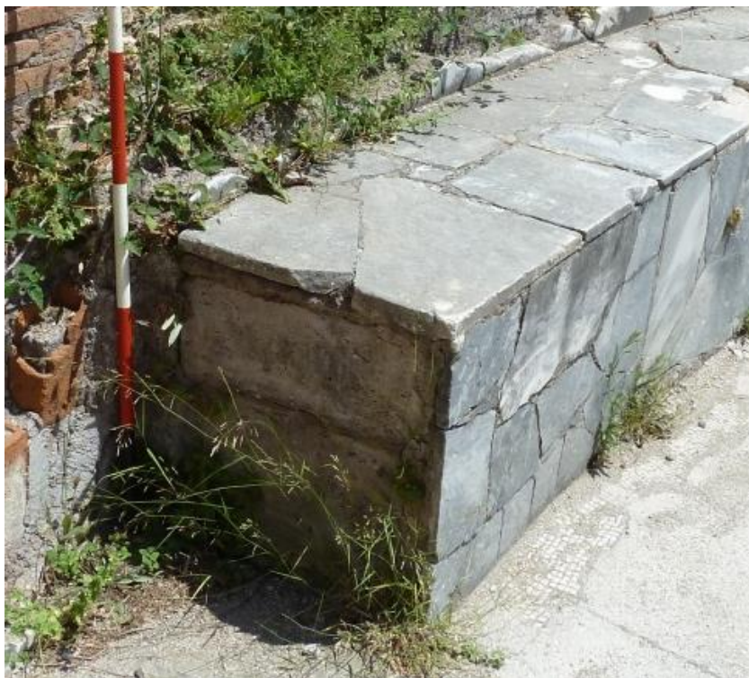
Figure 4-3: Marble Facing on Surface of Bench in Room 16
