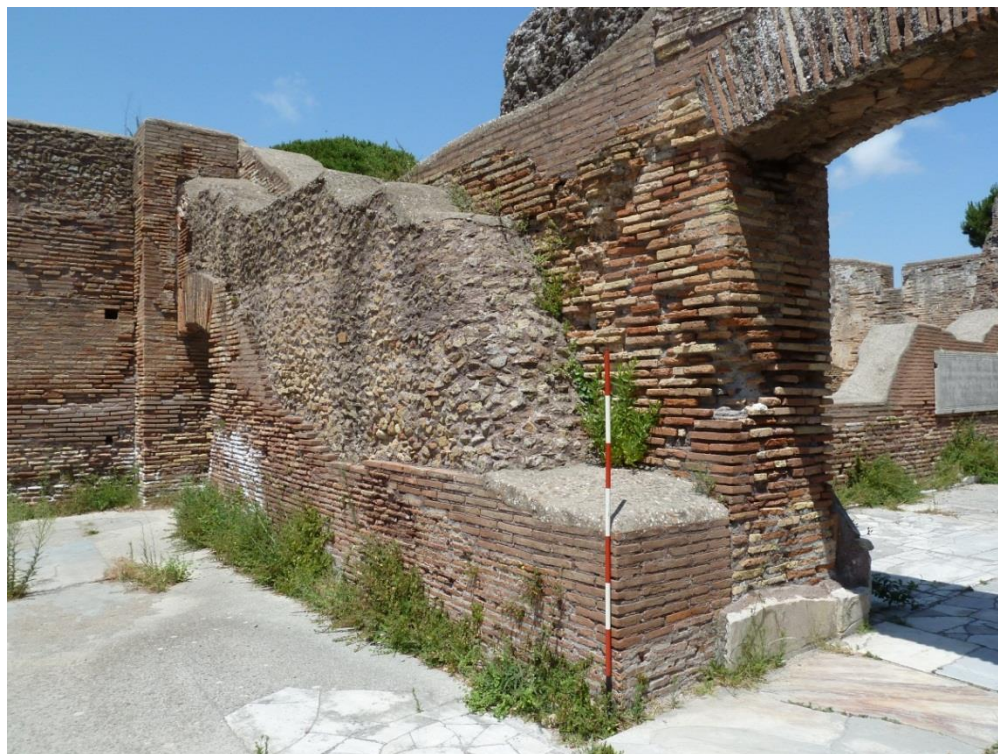
Figure 3-145: View Looking Northeast in Room 17 showing Double Walls and Door H
