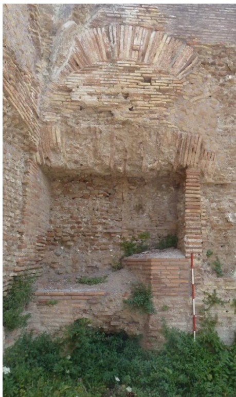
Figure 3-98: Blocked Door AI in Room 9
