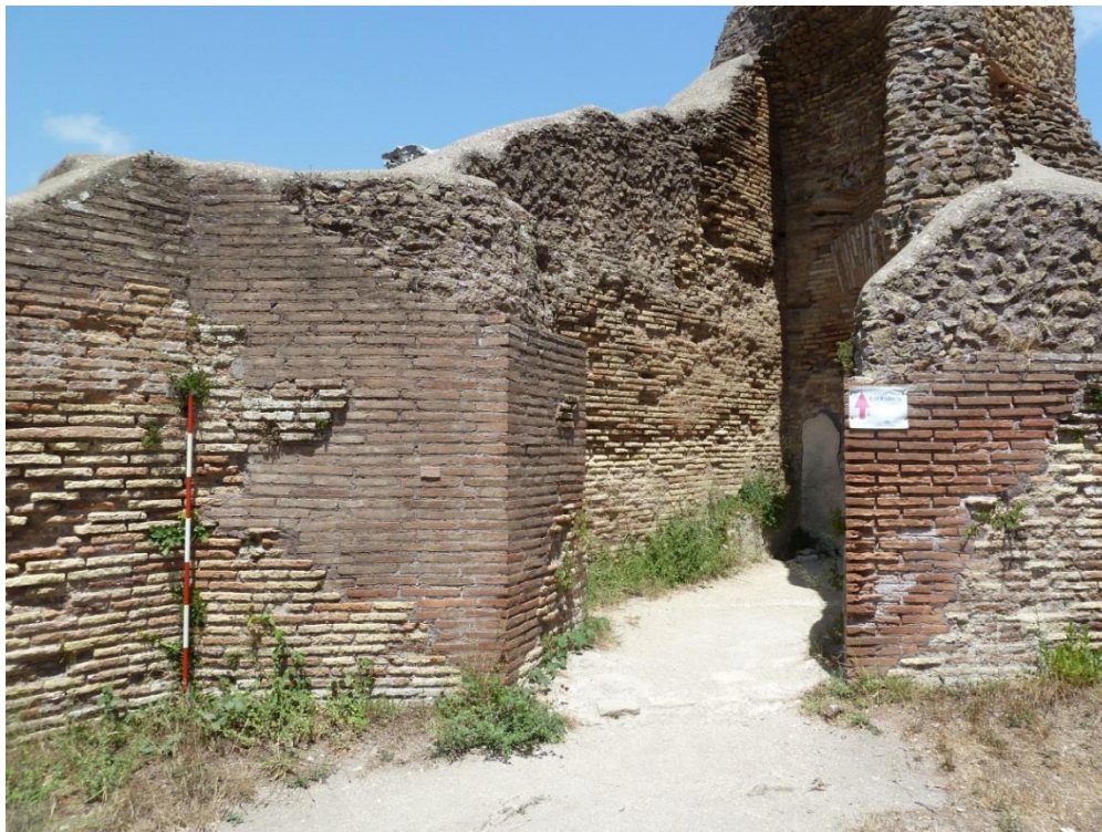
Figure 3-125: View Looking Northeast in Room 15 showing Door B and Room C
