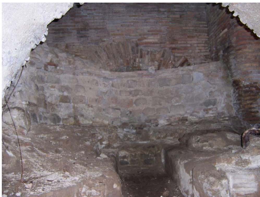
Figure 3-166: Furnace Opening for Room 19 East of Pool \gamma in Substructures
