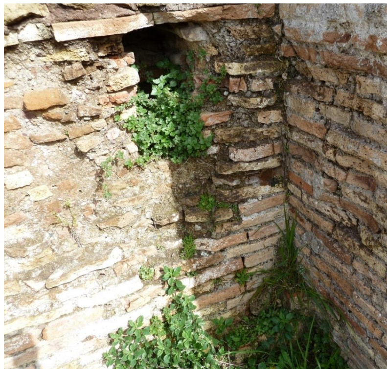
Figure 3-101: Opening in Wall b in Room 7
