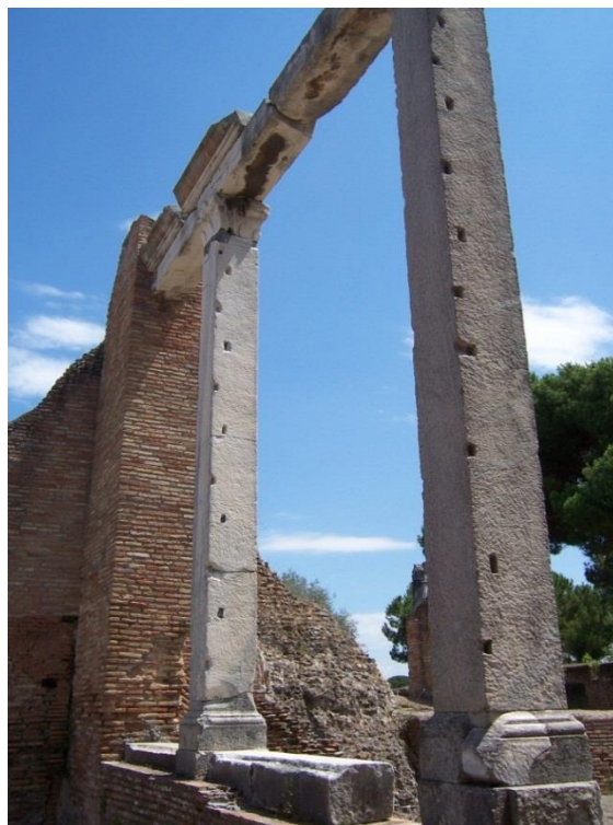
Figure 3-184: Pillars P1 and P2 in Room 18 showing Possible Evidence for Window Frames
