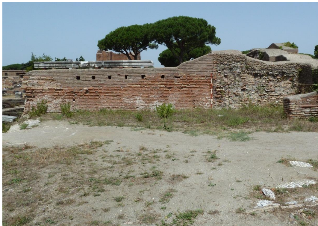
Figure 3-58: View Looking North in Room 1
