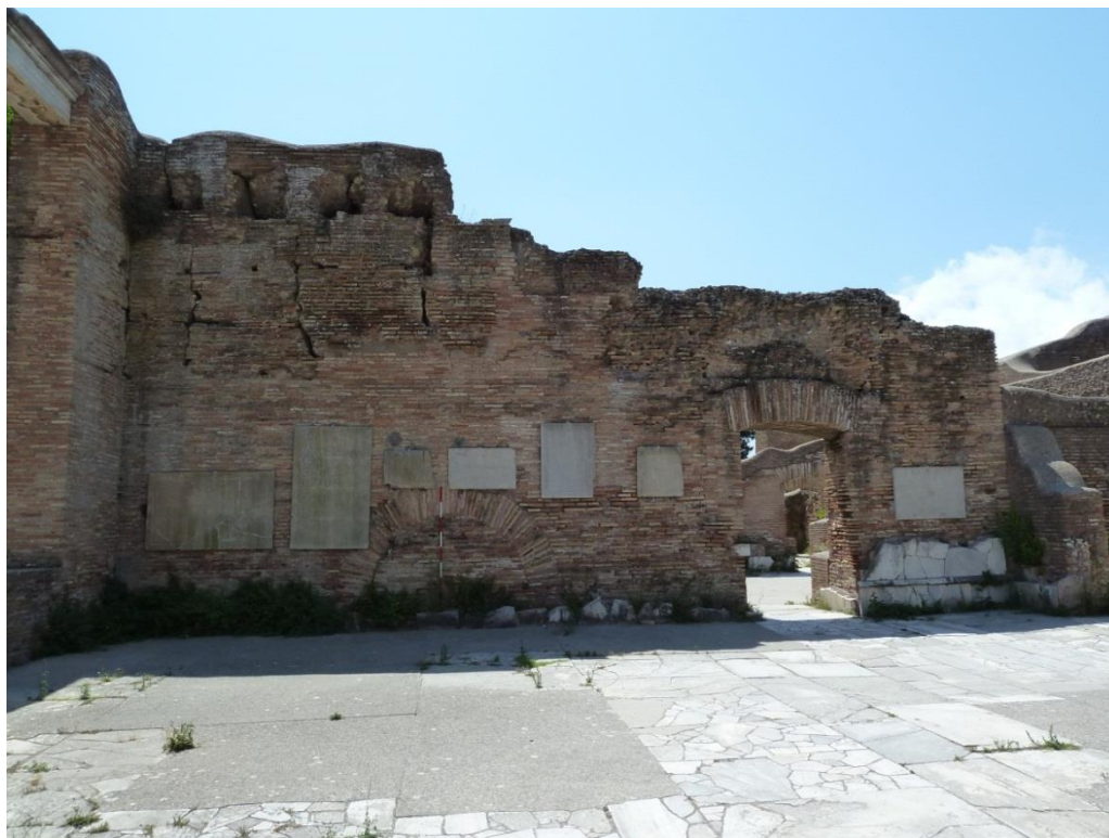
Figure 3-156: View Looking West in Room 18
