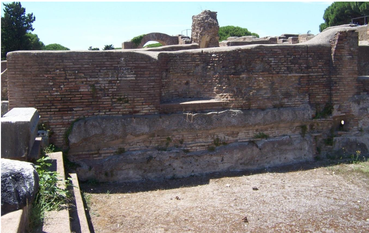
Figure 4-11: Wall c and Niche n2 showing Extra Layer of Brick Wall in Pool \delta in Room 6
