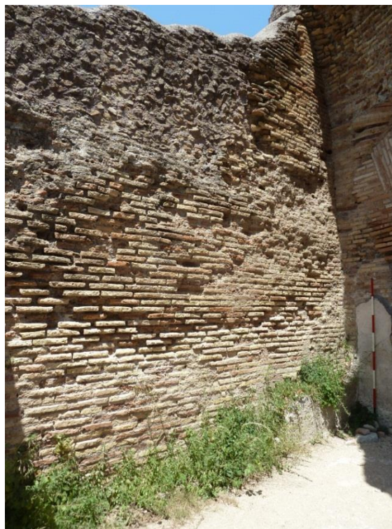
Figure 3-130: View Looking Northeast into Room C from Room 15
