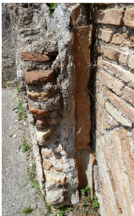
Figure 4-10: Wall c showing Extra Layer of Brick Wall in Pool \alpha in Room 19
