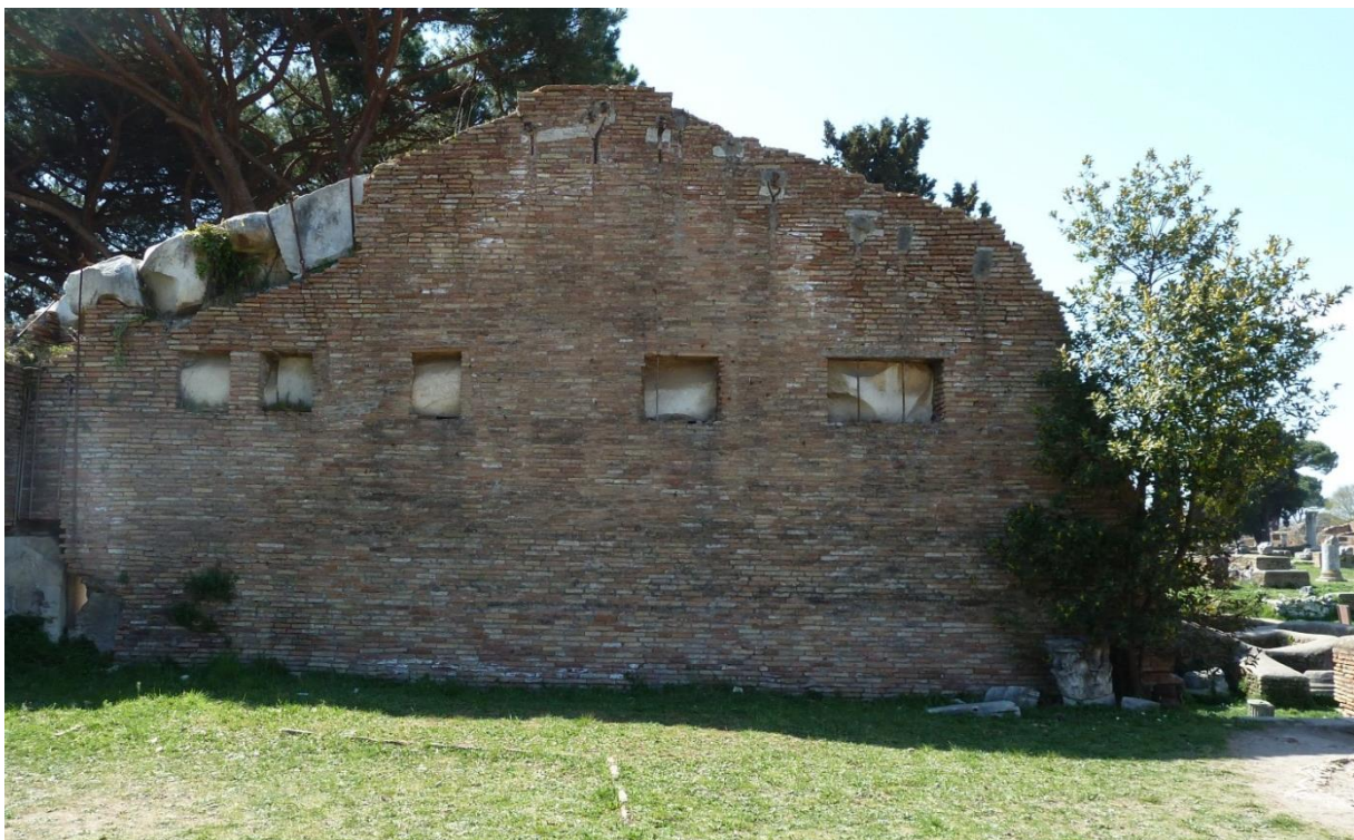
Figure 3-53: View Looking West in Room 1
