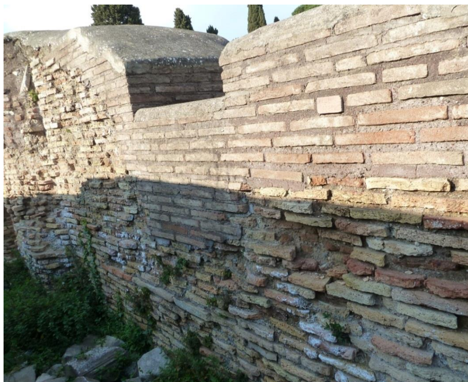
Figure 3-51: Possible Window in Eastern Wall of Room a2
