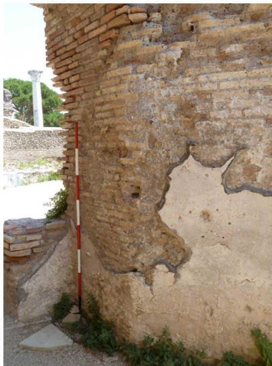
Figure 3-131: View Looking Southeast in Room C into Room 16
