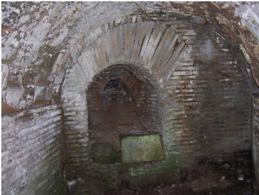
Figure 3-126: Furnace Opening for Room 15 in Substructures
