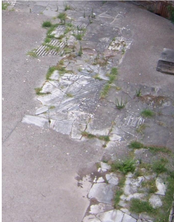
Figure 3-23: Pavement of Room 17 showing Reused Materials
