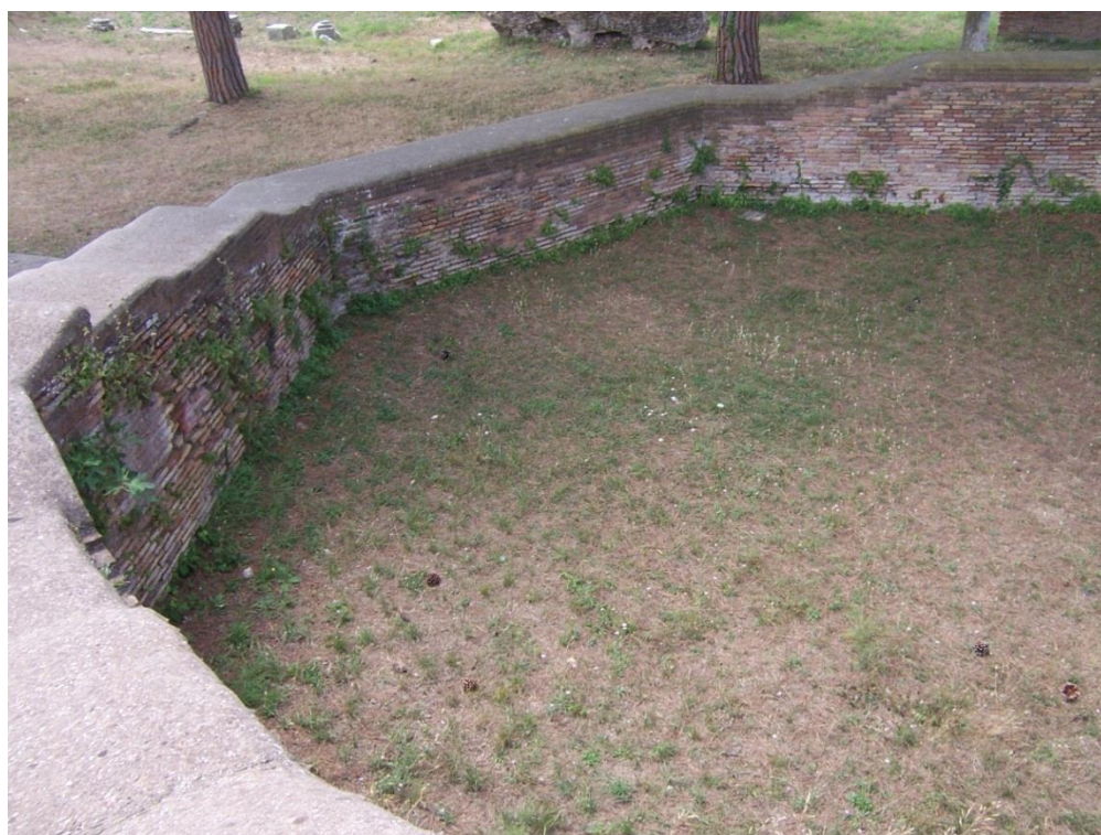
Figure 2-13: Heliocaminus (Room 15) Looking Southwest in the Terme del Foro, Ostia
