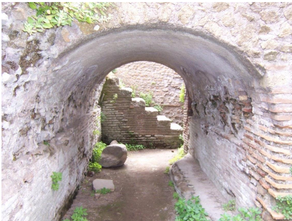
Figure 3-31: Staircase Leading to the Substructures below the Terme del Foro near Room 18
