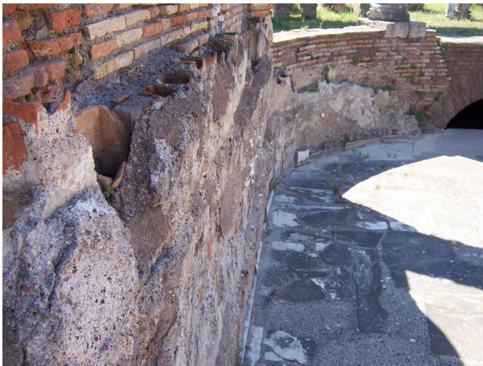
Figure 3-161: View Looking South in Pool \gamma in Room 19 showing Tubuli and Pavement
