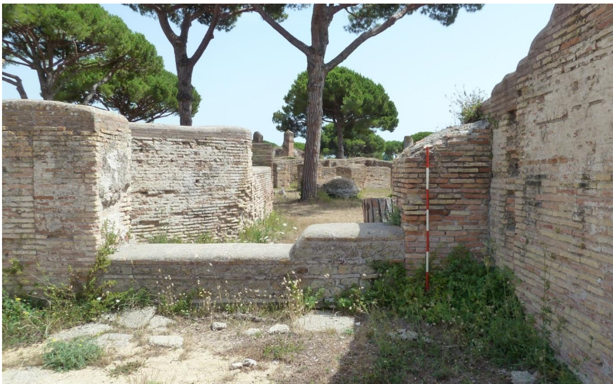
Figure 3-77: Walls n, o, p and q and Door Y in Room 2
