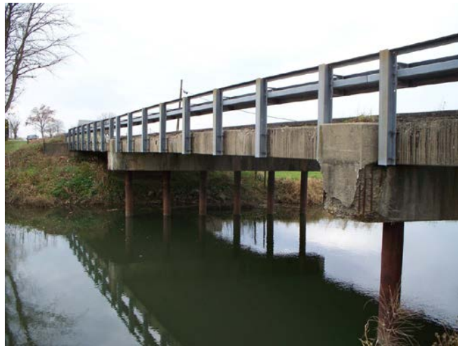
Figure 17 - Phase II - Center Span (Steinberg, 2011)
