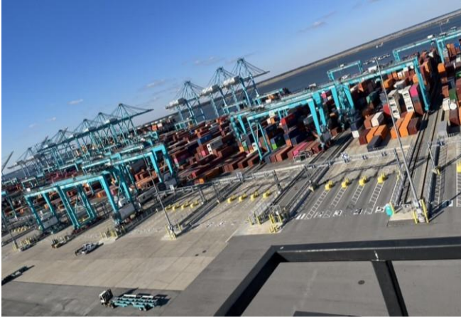
Fig. 4. Ship-to-Shore (STS) Cranes at a Maritime Container Port
