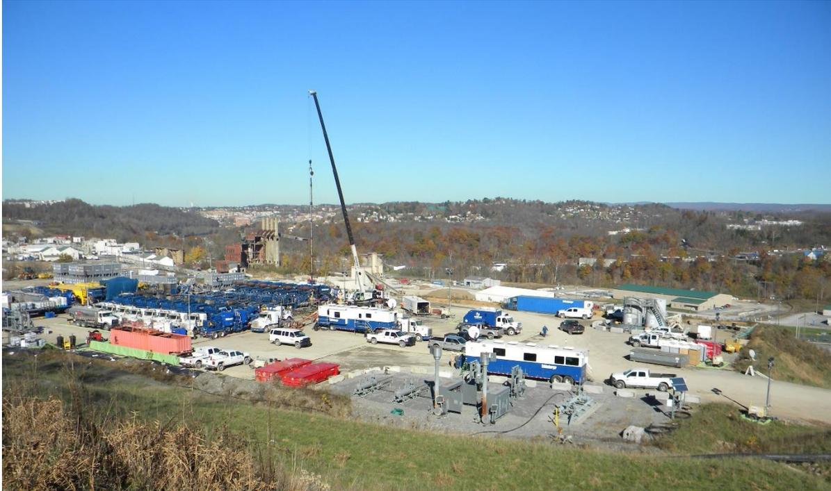
**Figure 1-2: Marcellus wellhead showing support equipment for drilling and fracturing multiple wells at a single well site.**
