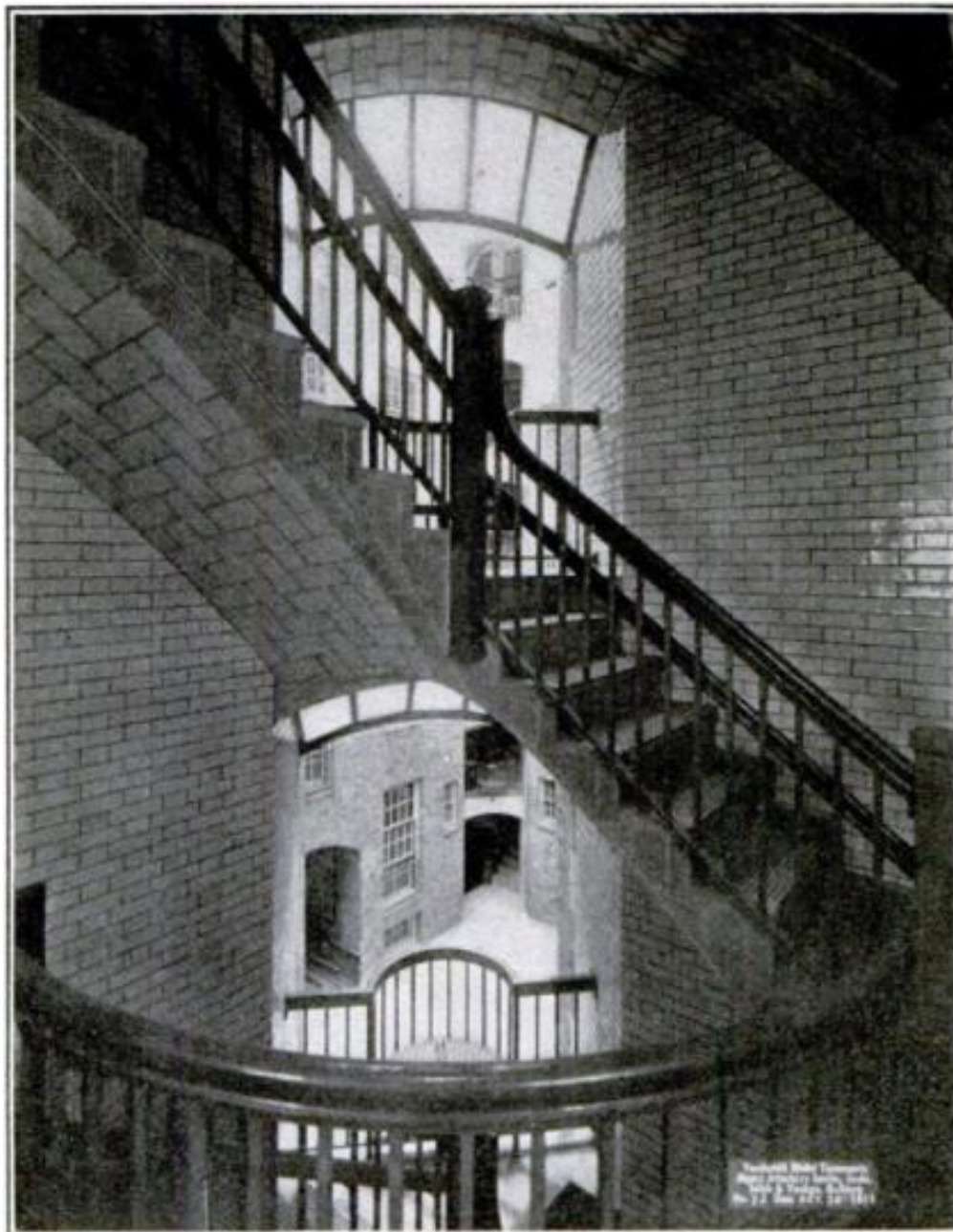
Figure 18: Stairs in the Open Stair tenement. From: Jonathan A. Rawson. "Modern Tenement Houses." Popular Science Monthly , February (1912): 193.
