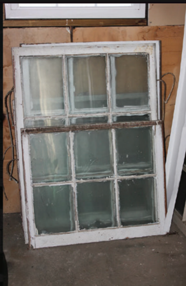
Image 3: Possible original wooden 6x6 double-hung sash window in storage, St. Johns School, Albemarle County, Virginia. Photograph by Hannah Glatt. January 17, 2017.
