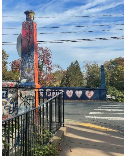
Fig. 3.2.2. Beta Bridge at UVA, column view
