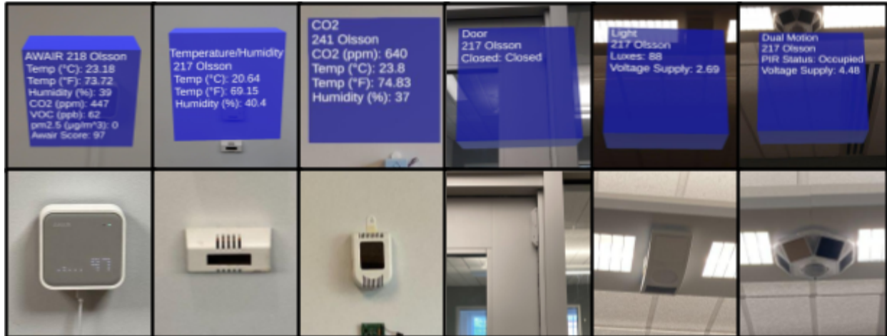
Figure 1: Sensor and Hologram Types (from left to right: Awair sensor, temperature and humidity sensor, CO2 sensor, door sensor, light level sensor, and dual motion sensor)
