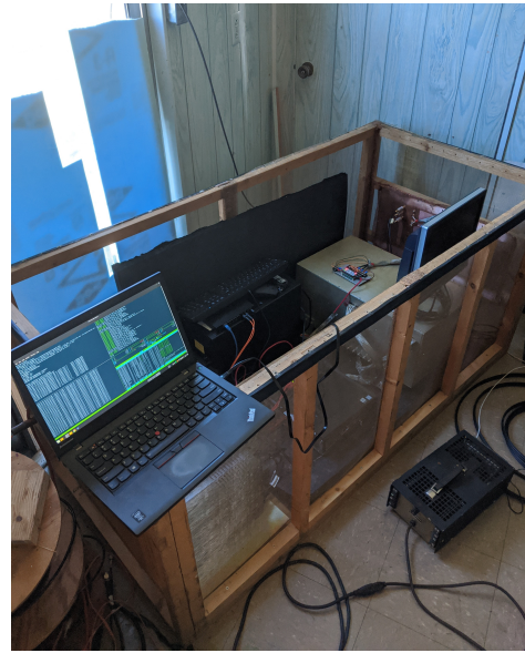
(b) Deploying backend in the GBO 45'-Telescope Trailer
