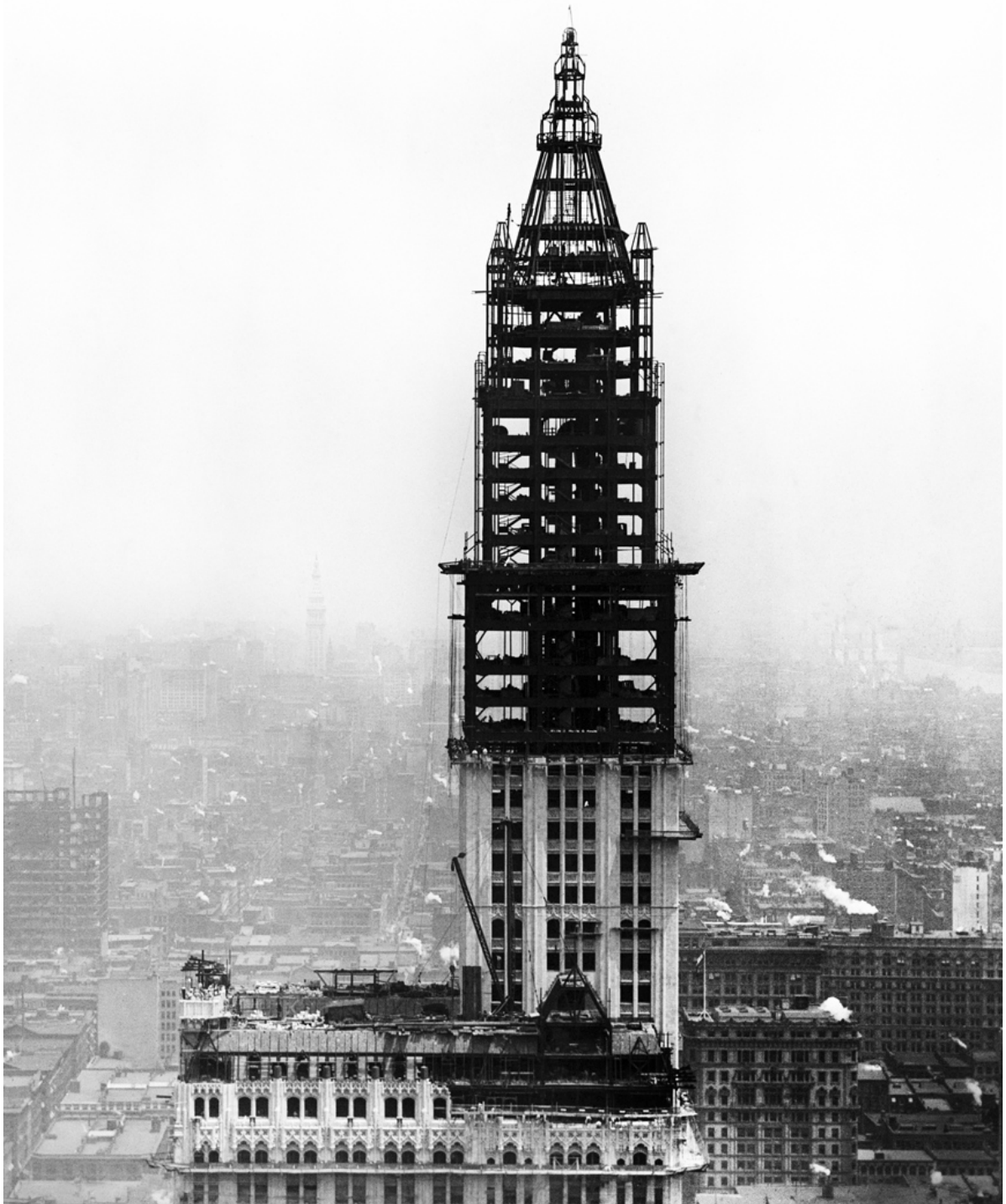
Figure 4. Woolworth Building under construction, exhibiting the steel frame. c. 1912. Bain News Service, Library of Congress.
