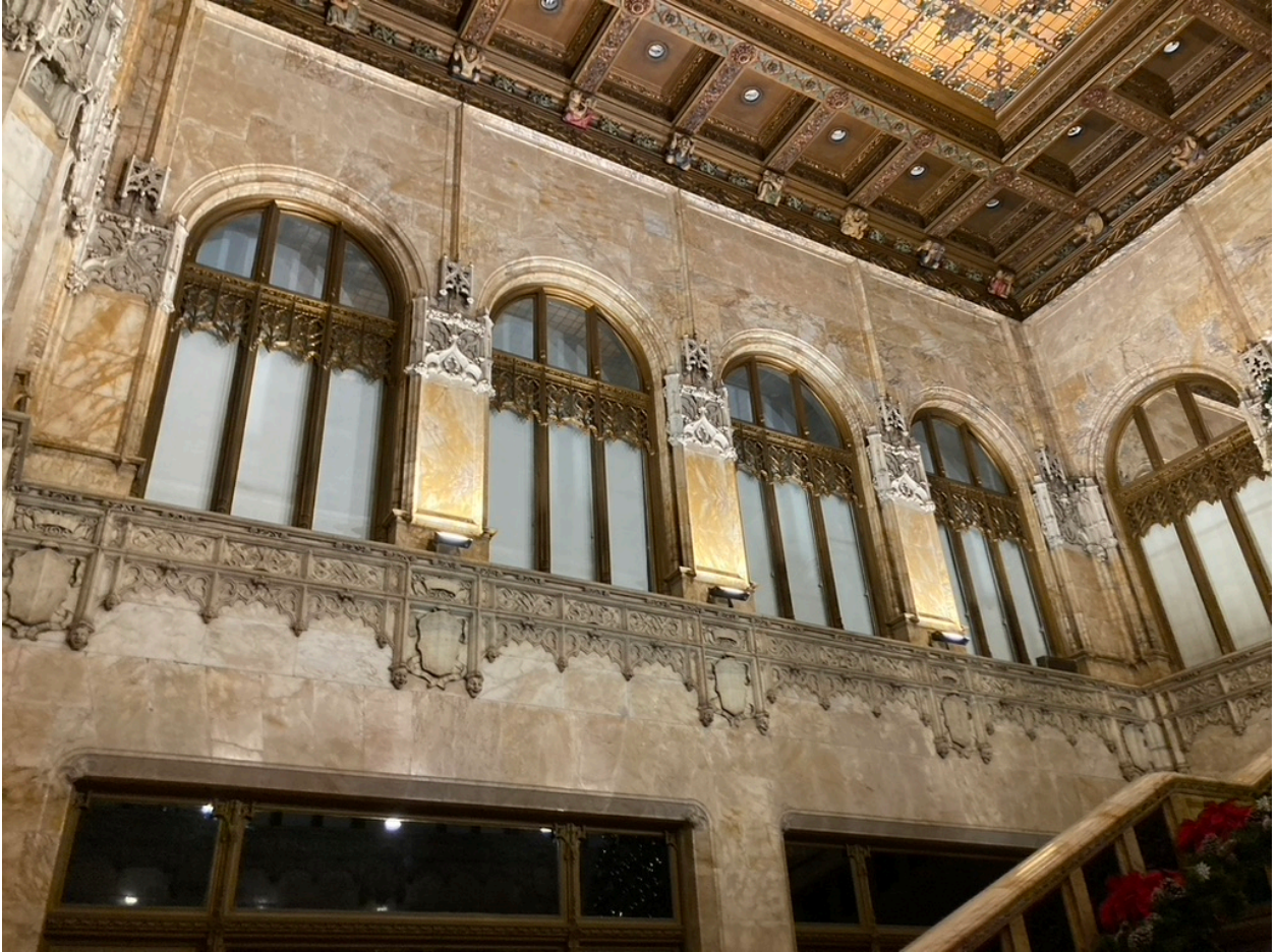
Figure 25. Detail of stone tracery profiles along the Marble Hall. Note the continuation of the tracery across the windows using metalwork. Photograph by author, December 2022.
