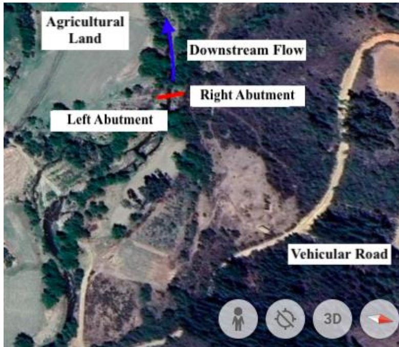
Figure 2. Aerial view of bridge site
