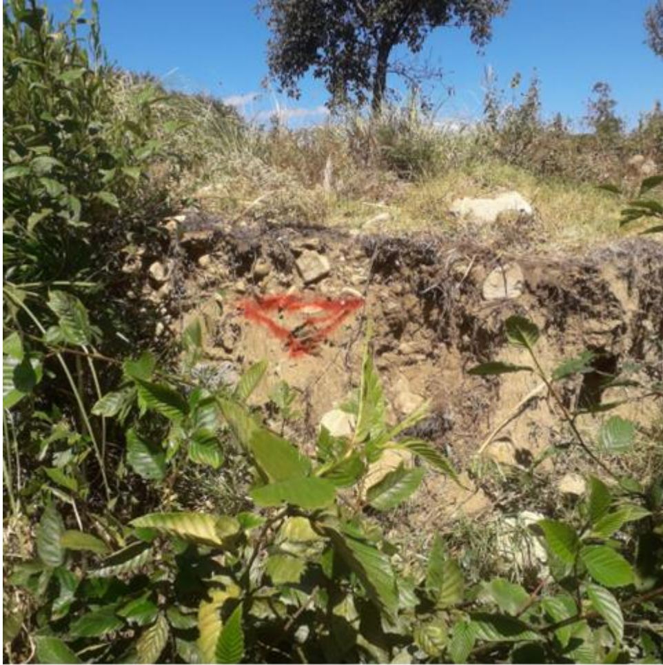
Figure 7. High-water line marking
