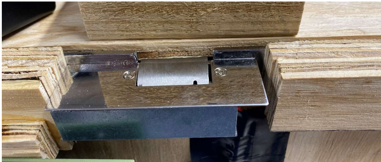
Figure 52 Front-View of Package Box Locking Mechanism
