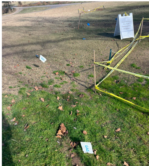
Figure 14: Flags showing utilities near head cut and across stormwater conveyance
