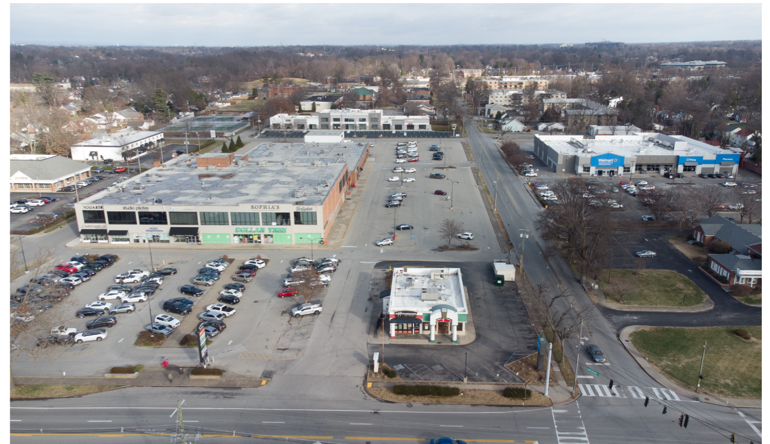
20. Existing Site Conditions
