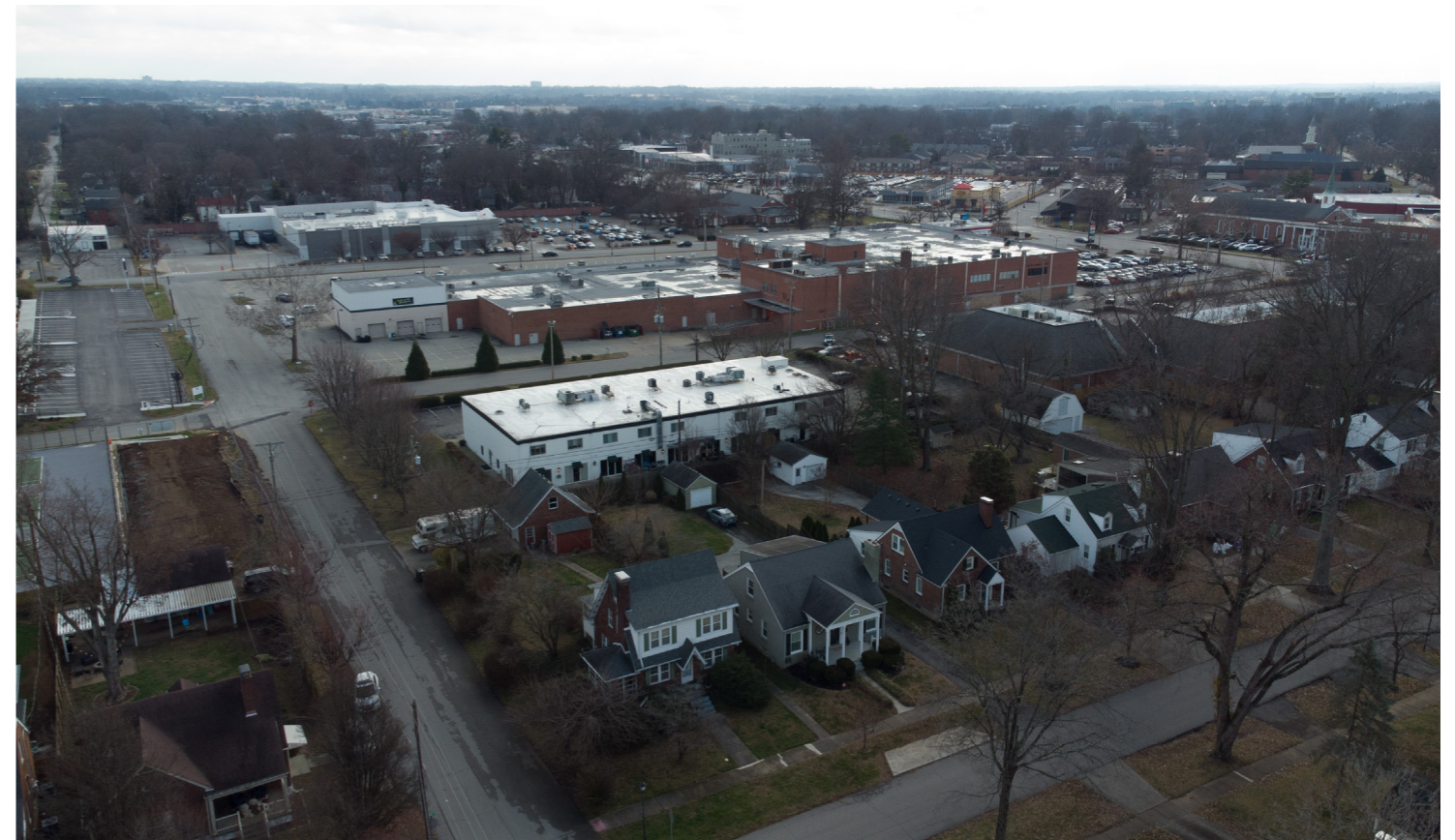
18. Existing Site Conditions
