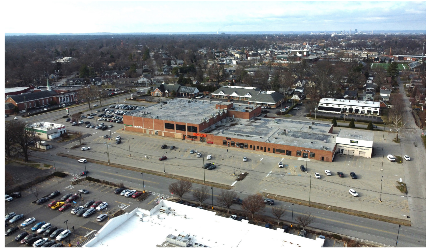
17. Existing Site Conditions
