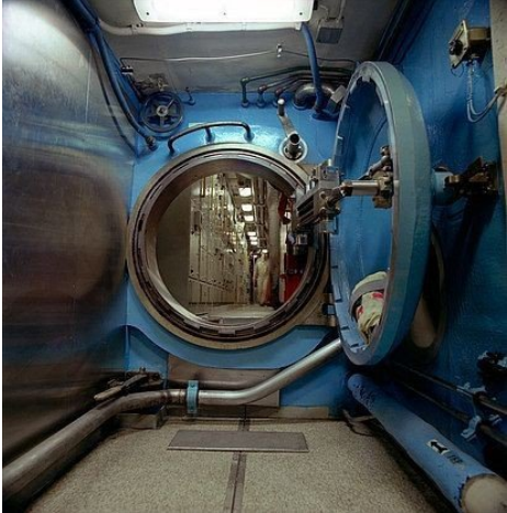
Figure 2: Image of Submarine Watertight Door.
