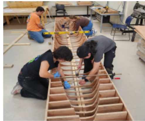
Figure 2. Mold Construction
