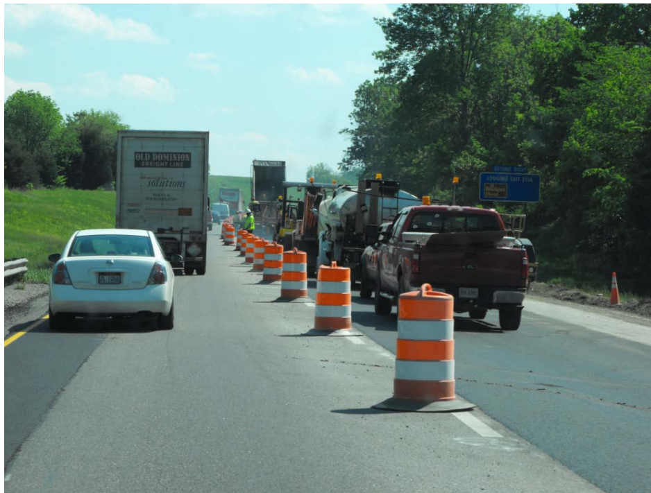
Figure 11. Slow-moving traffic through I-81 work zone adjacent to construction activity.
