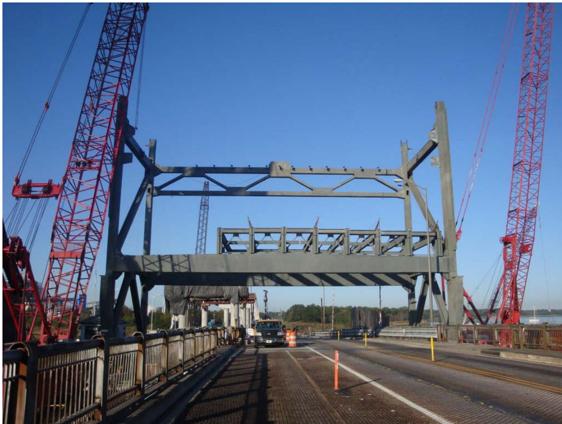
Figure 17. Work zone setup across Gilmerton Bridge.
