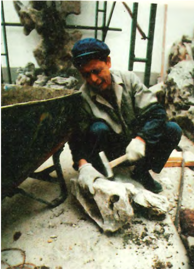
Fig 1.10. Workman shaped pieces of Taihu rock at the construction site. Image from Henry Mitchell, "An Oriental Garden Grows, Elegantly in Mid-Manhattan," Smithsonian 12, no. 4 (July 1981), 69.
