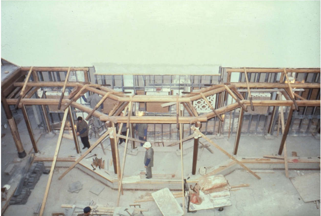
Fig 1.6. Pillar structures of the winding walkway/covered zig-zag corridor ( qu lang ) at Astor Court. In traditional Chinese architecture, the pillars not the walls, support the entire weight of the finished building. Image: Astor Chinese Garden Court, construction, view 7 , March 10, 1980, slides (photographs), 2 x 2 in., the Department of Asian Art at The Metropolitan Museum of Art (New York, N.Y.), accessed January 31, 2021, https://libmma.contentdm.oclc.org/digital/collection/p16028coll14/id/2373
