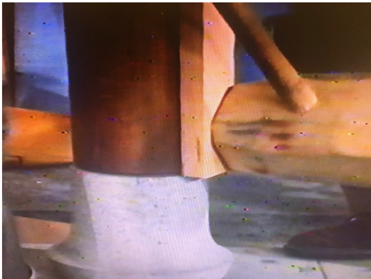
Fig 1.7. Wooden mallet used for the alignment of pillars. Image screenshotted from Gene Searchinger, Ming Garden , Video; VHS (Mass: Home Vision, 1983).
