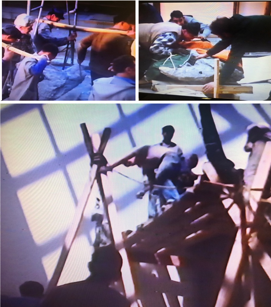
Fig 1.12 – 1.14. Traditional methods of rockery construction. Wooden tripods were used following the traditional method to shift the great rocks, each weighing a ton or so. Images screenshotted from Gene Searchinger, Ming Garden , Video; VHS (Mass: Home Vision, 1983).
